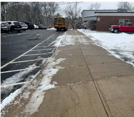
Site lacks separate bus/car drop-offs and sufficient parking
