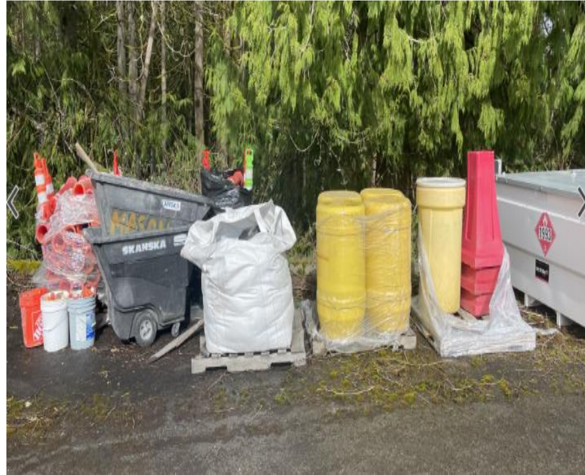
Construction support materials arriving on the site
