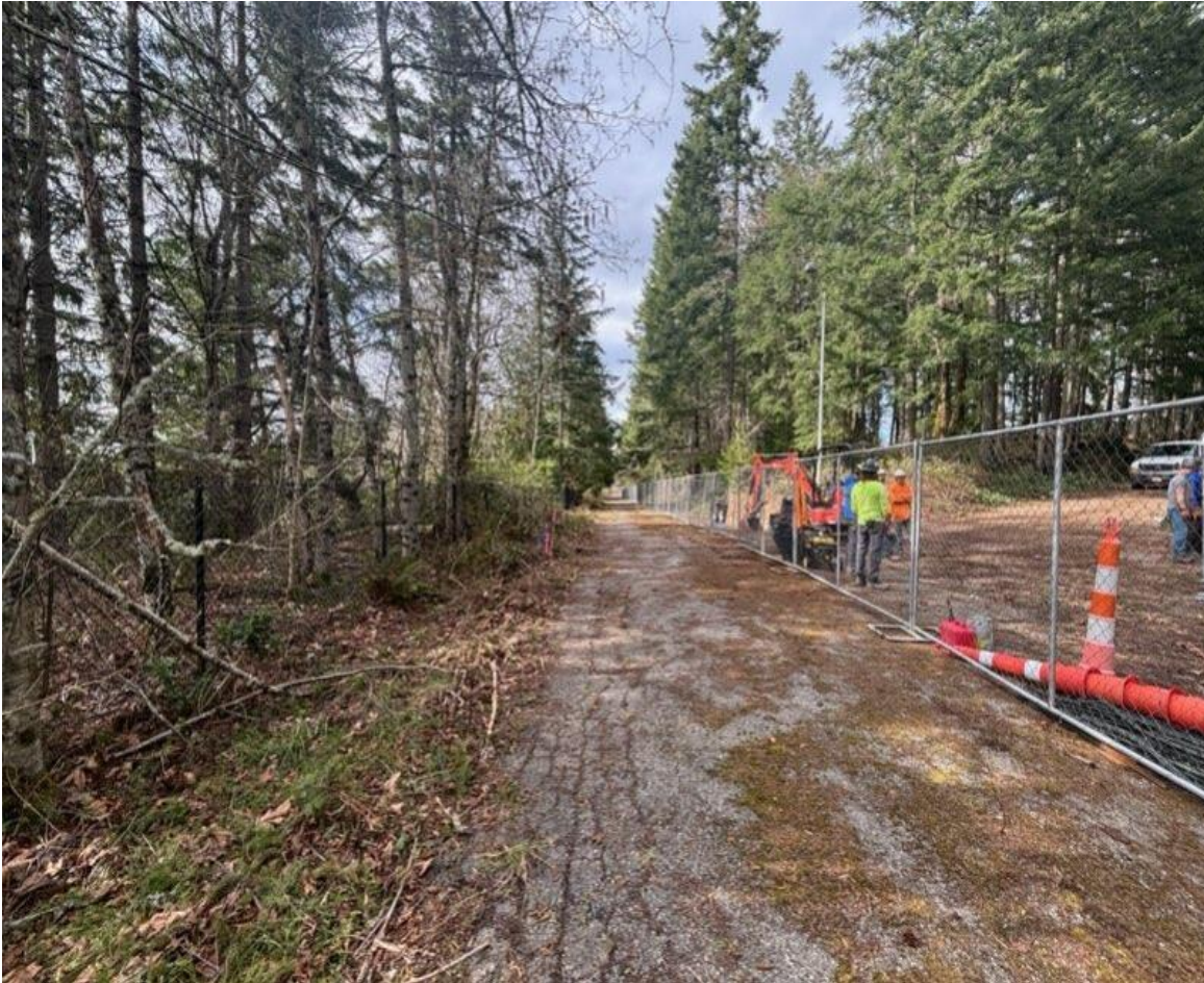
Perimeter construction fencing at south drive installed
