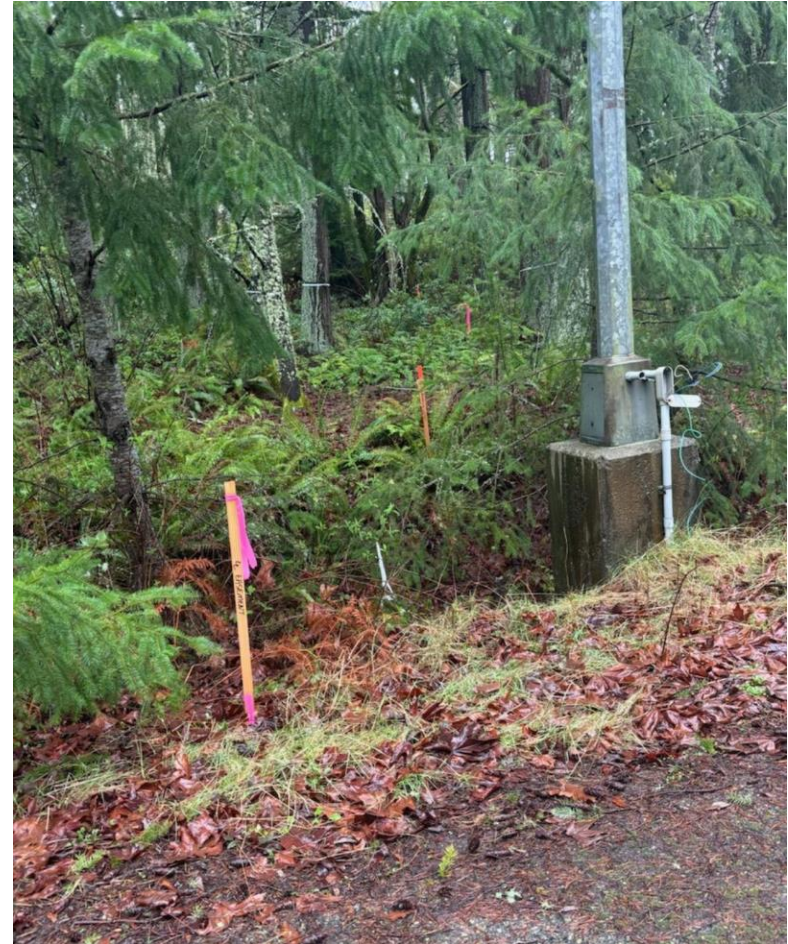
Clearing limits being surveyed and staked
