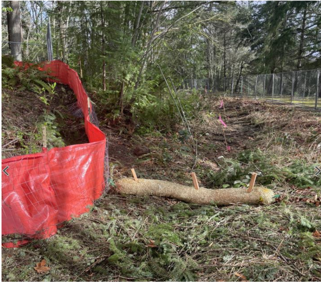
Temporary Erosion Sediment Control (TESC) measures being installed
