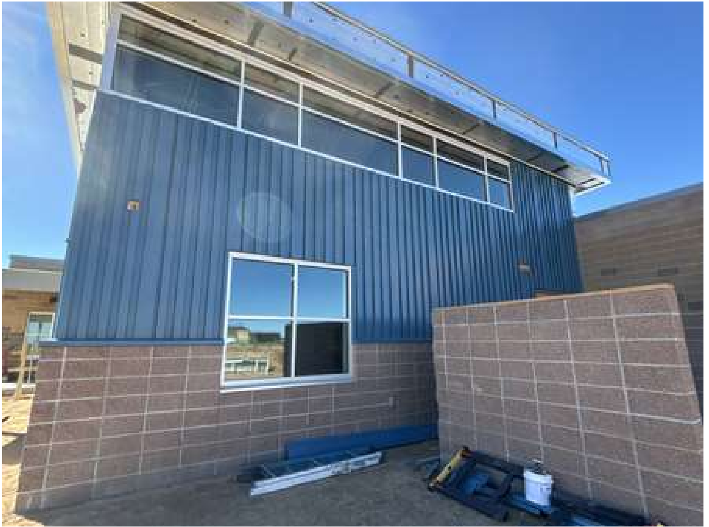
New Metal Siding
