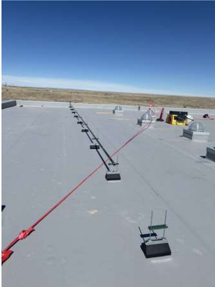
Roof on Addition
