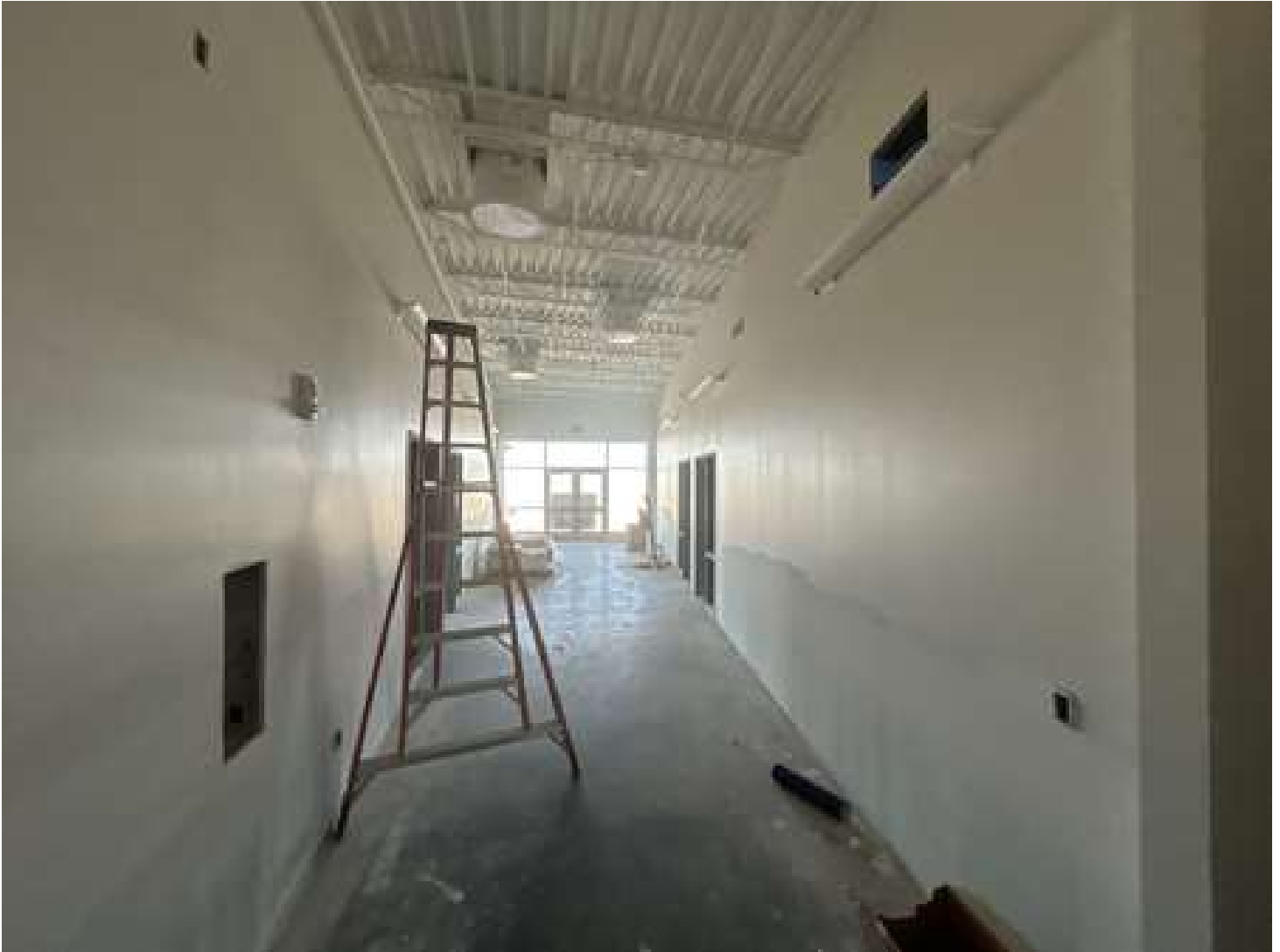
Hallway to Classrooms in Addition
