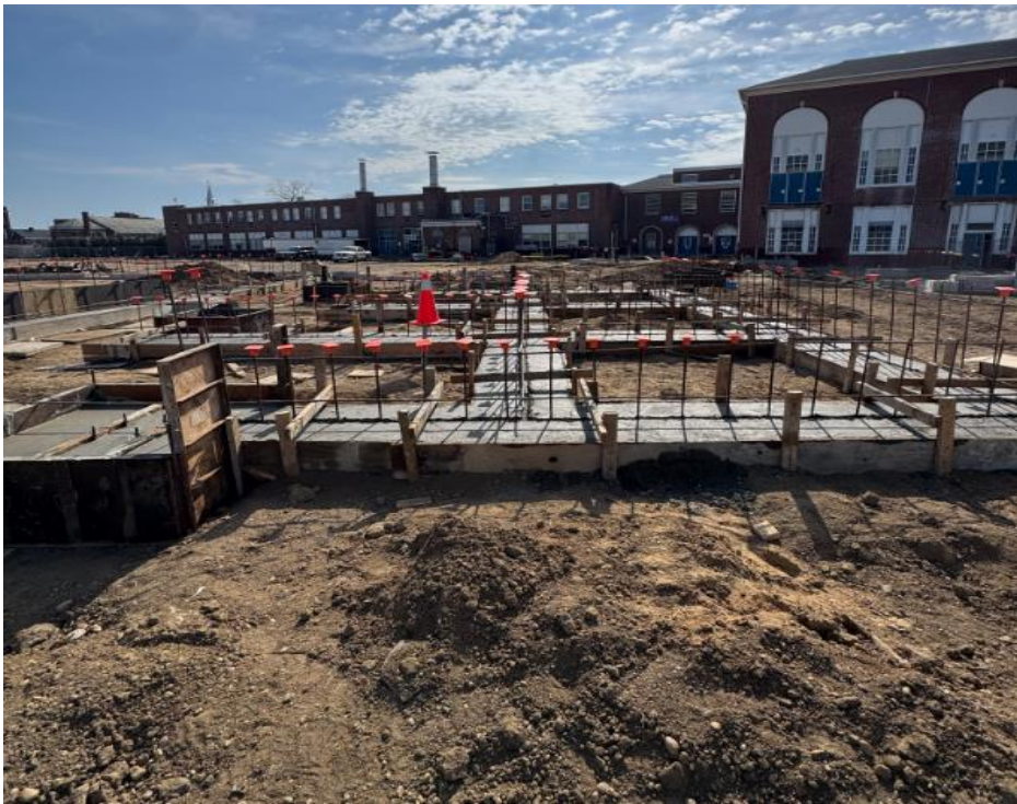
Hempstead ABGS MS – Interior Piers and Walls
