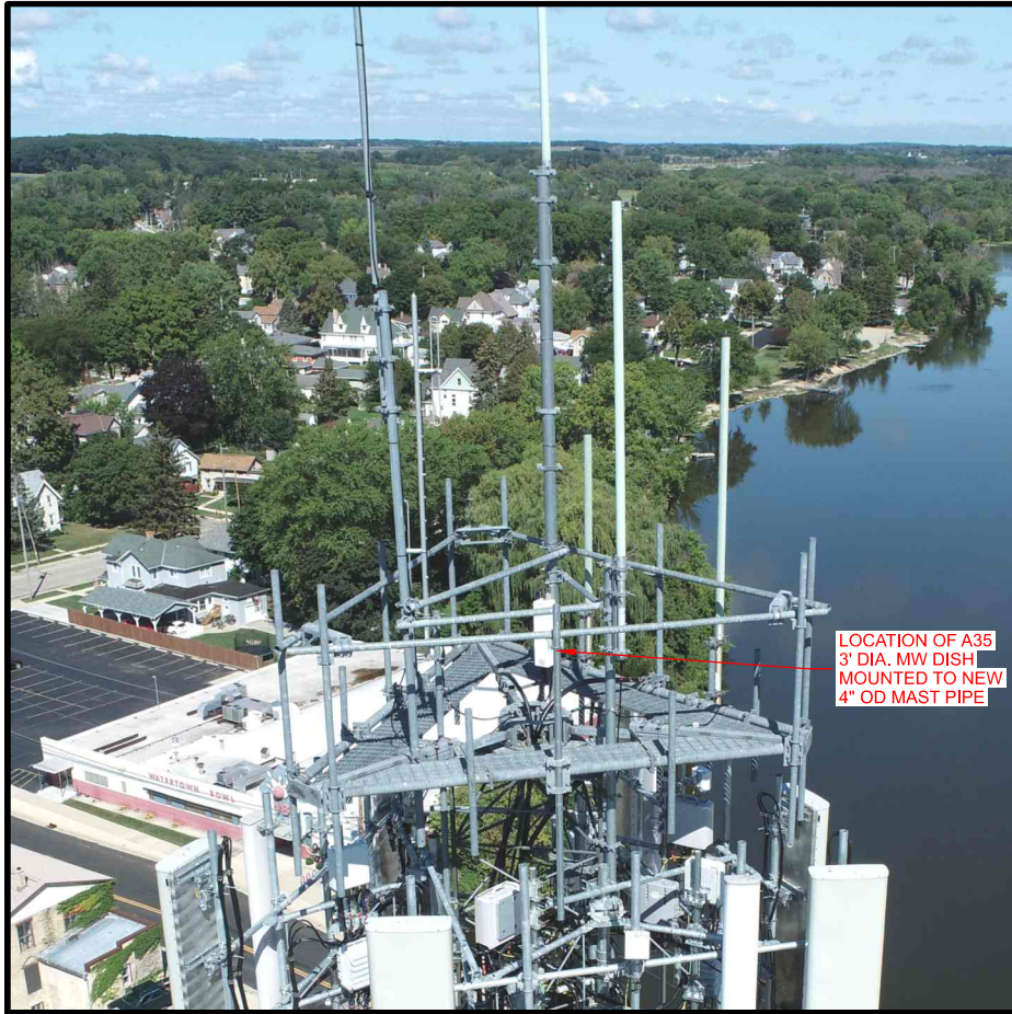
A EXISTING PLATFORM - FACE B-C
