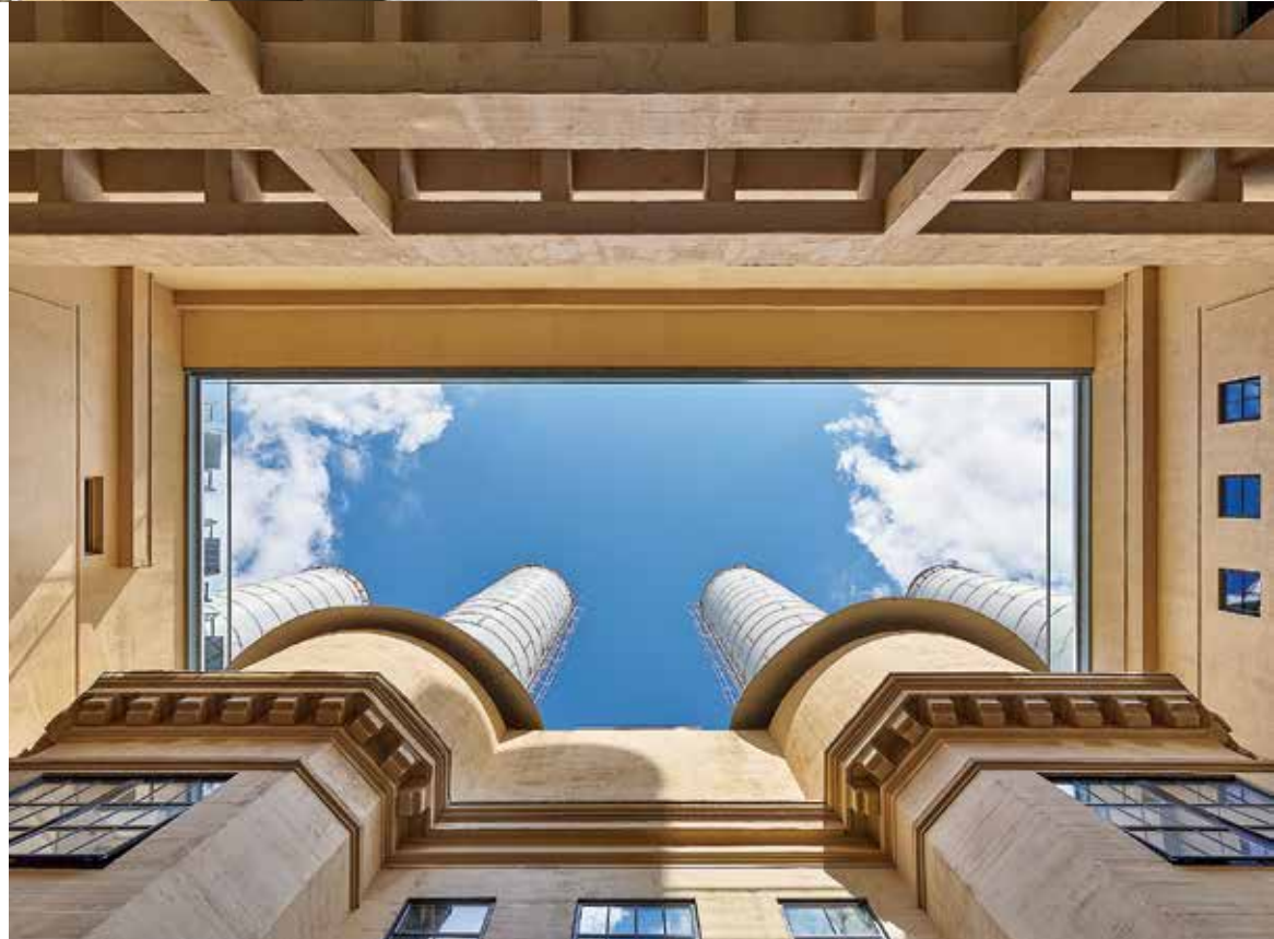
Right: Exhaust stacks looking skyward JEFFREY TOTARO
