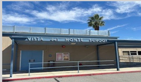
View of front of school - MPR
