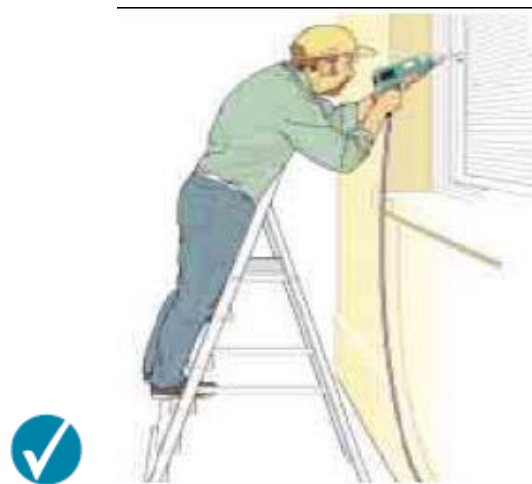
Correct – steps facing work activity
