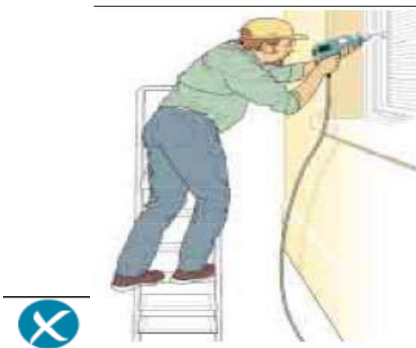
Incorrect – steps side on to work activity
