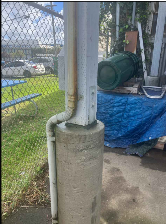
PHOTO 2: EXISTING RAINWATER LEADER
