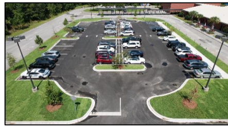
E.B. Ellington Parking Renovations
