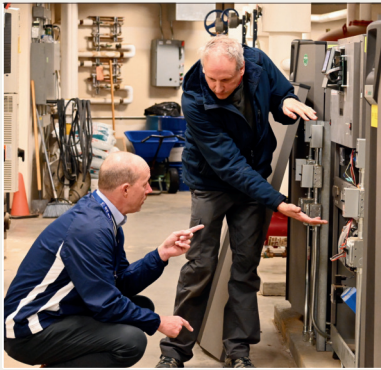
District HVAC journeyman Rod McMichael shows Superintendent Ben Ferney some of the equipment he maintains and services every day.
