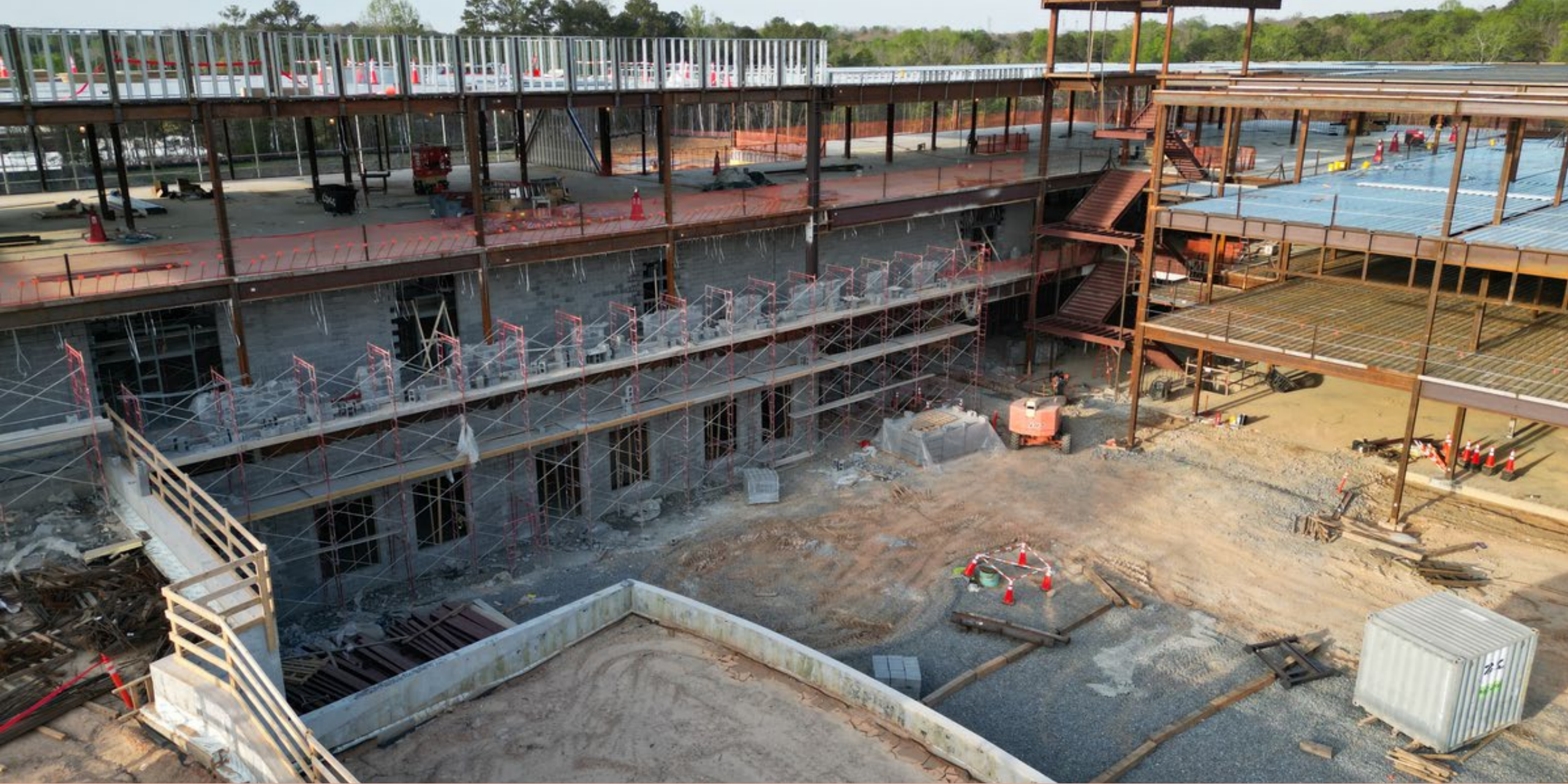
Exterior Framing and Interior CMU work
