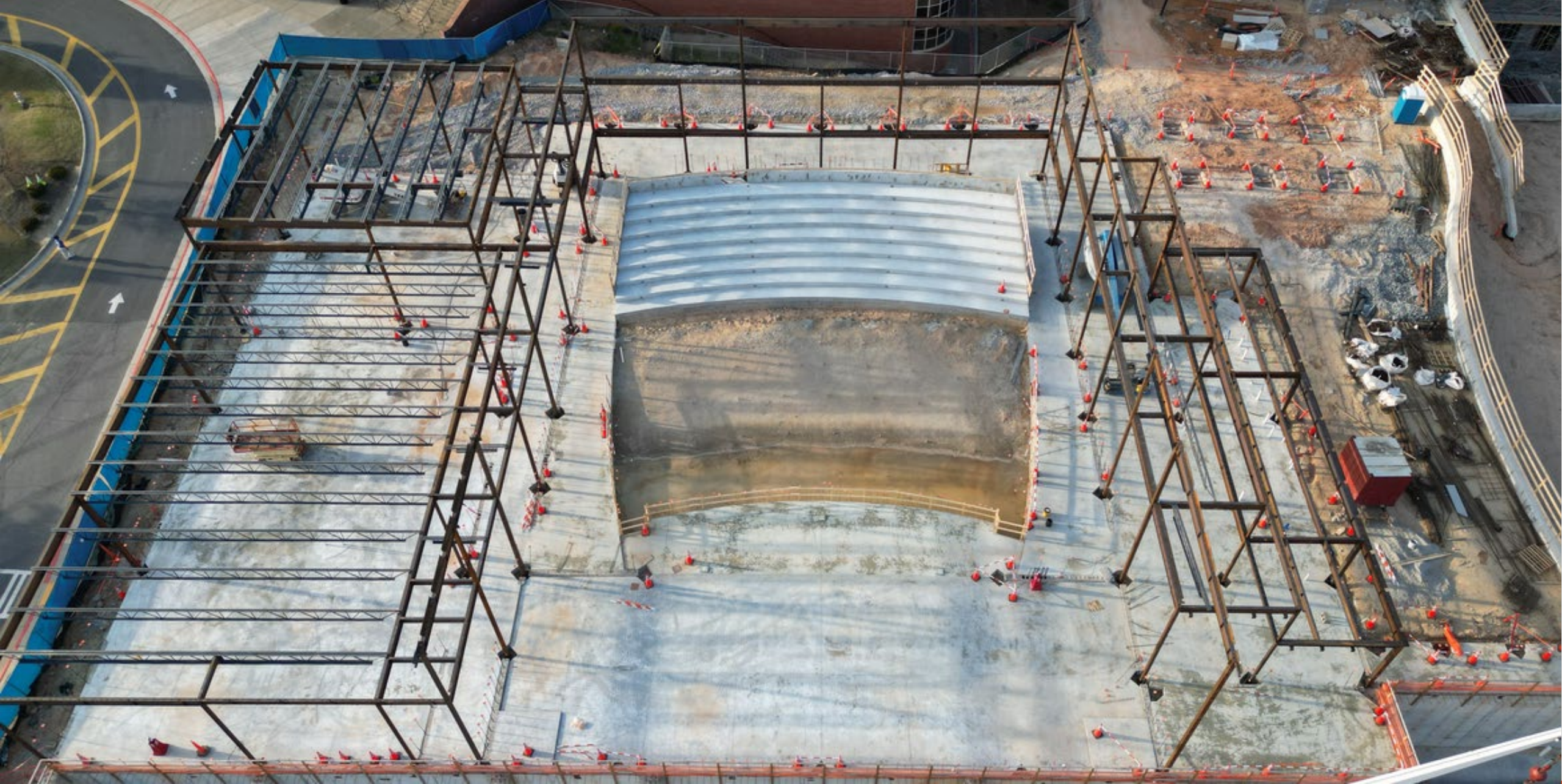
Area 8- Auditorium Steel Erection in Progress
