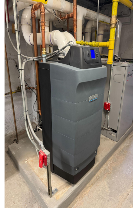
Boiler Replacement at Watchung
