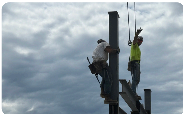
Skilled members of Ironworkers 417, began building the frame of the brand-new security vestibule.
