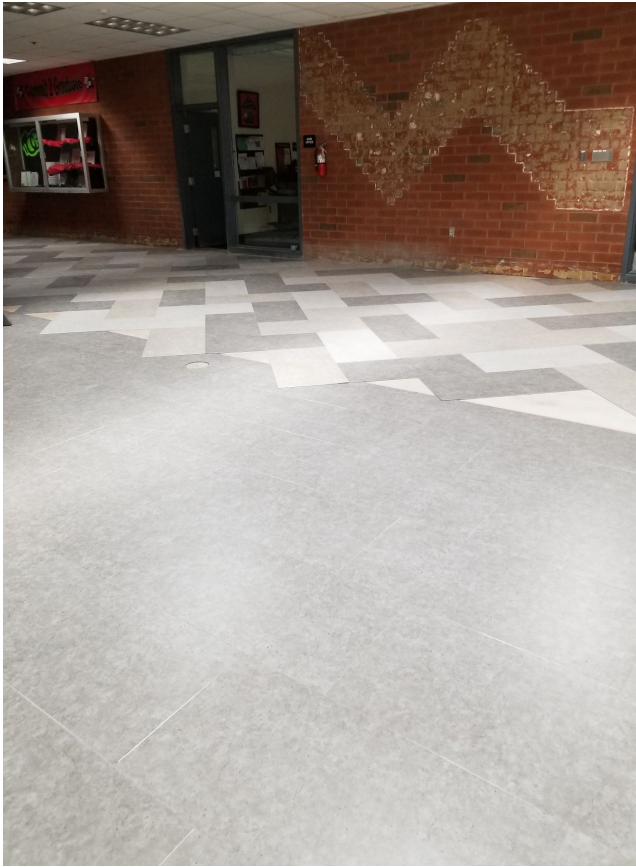
BPHS Cafe Flooring Replacement
