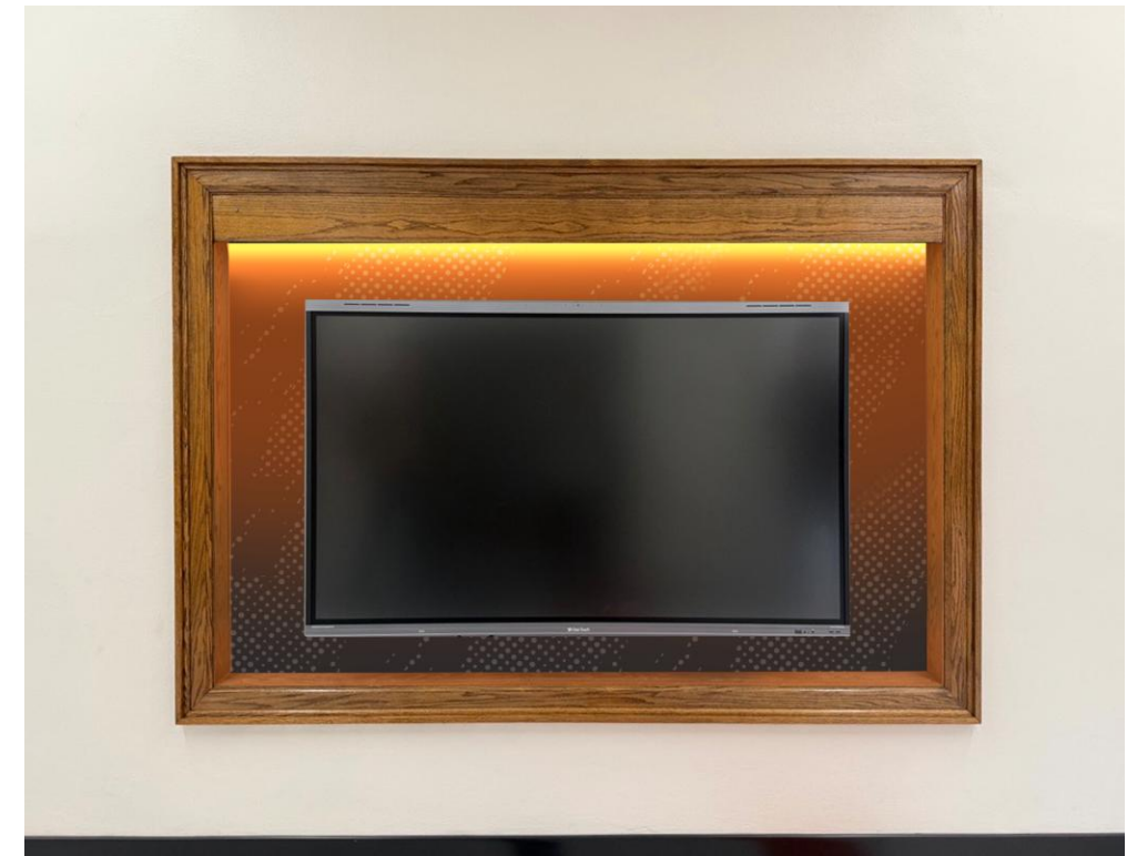
Option 3 Rear panel covered with digital graphic, accent LED color light concealed inside upper frame
