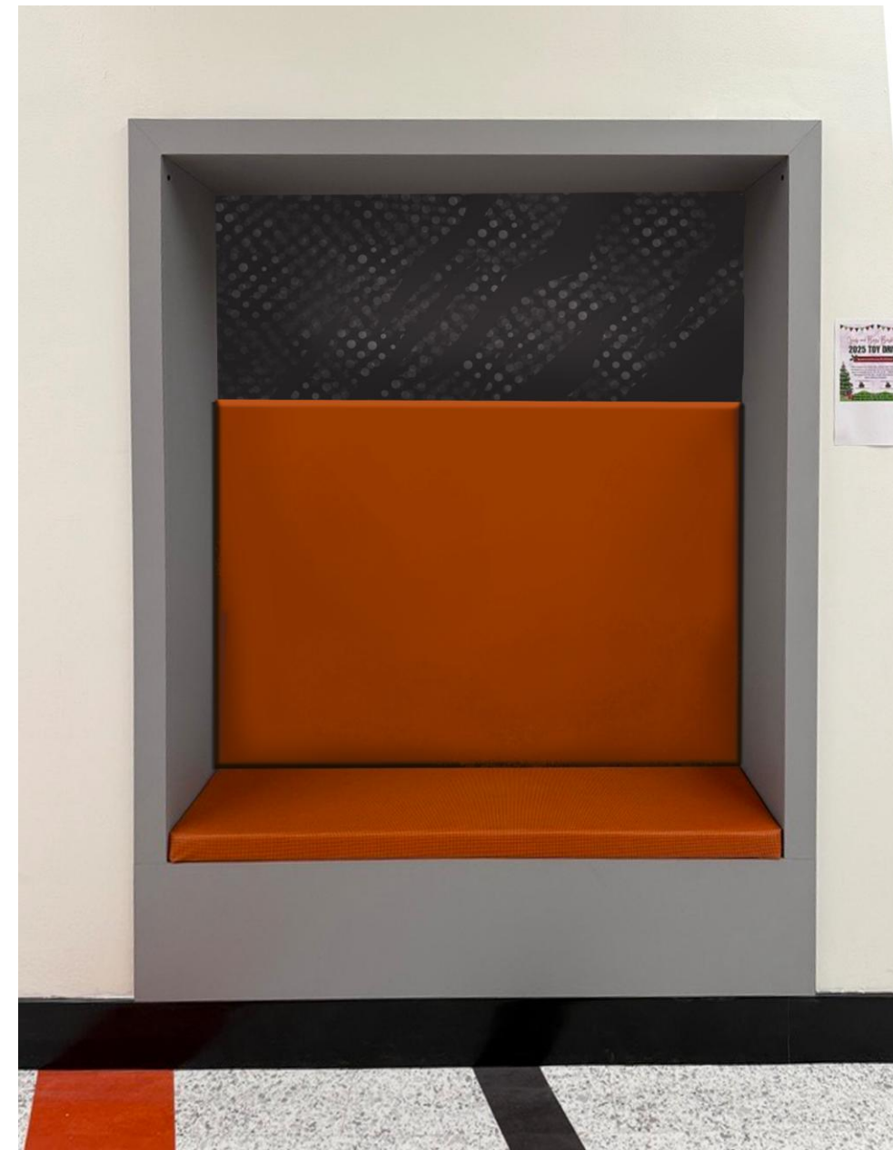
Option 3 Rear panel covered with digital graphic and partial height back cushion
