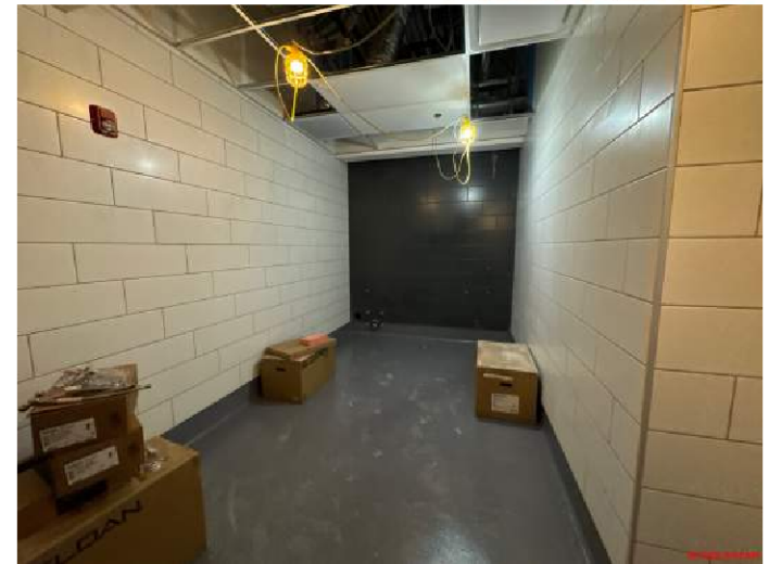
Bathroom Tile / Epoxy Flooring
