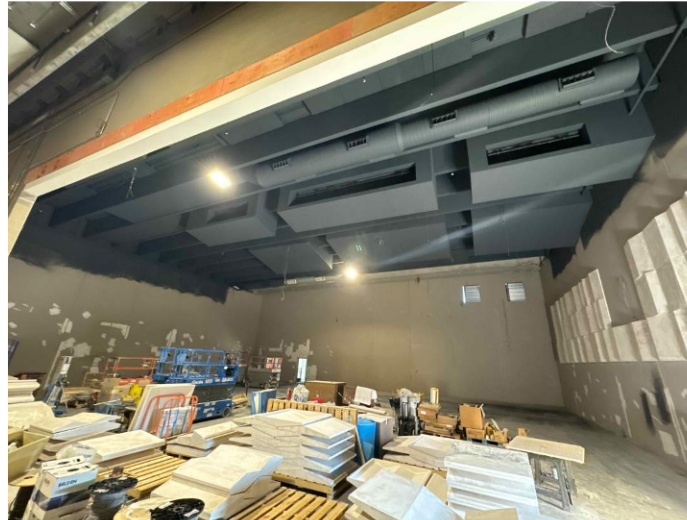
SVMS - Ceiling Dryfall & Walls Primed
