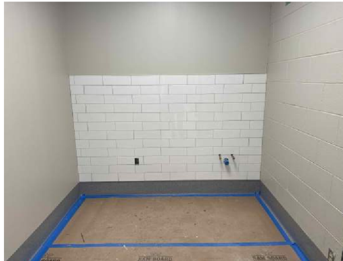
Restroom/Changing room wall tile
