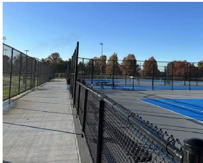
East Concourse Looking South
