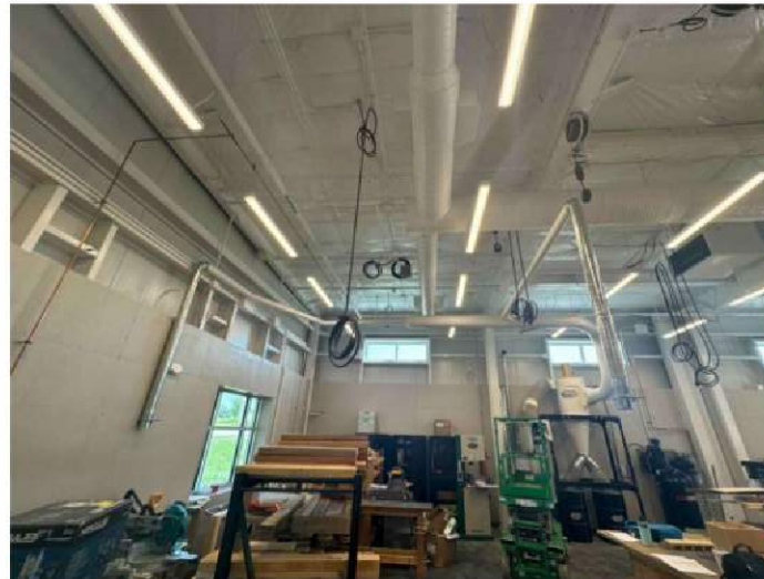
Dust Collection Install Complete in Shop
