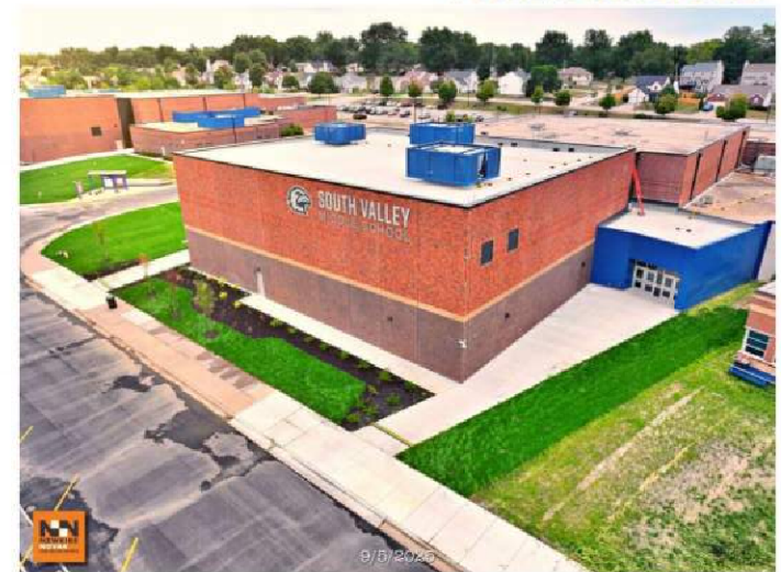
SVMS Exterior View
