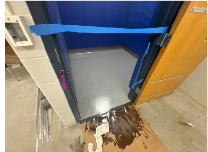
Safe Room with new epoxy floors
