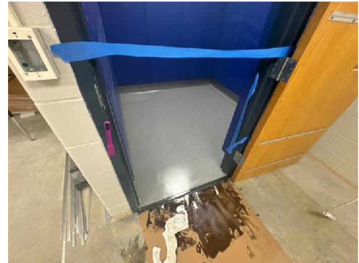
Safe Room with new epoxy floors
