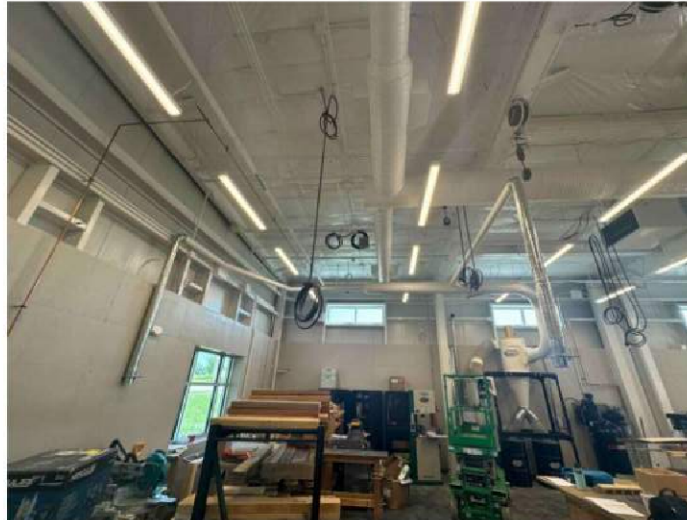
Dust Collection Install Complete in Shop
