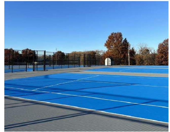
North Courts Looking Southwest
