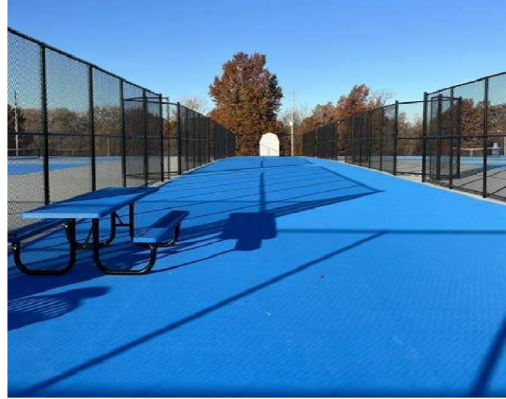
Center Spectator Concourse Looking West
