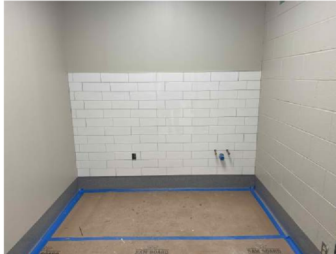
Restroom/Changing room wall tile
