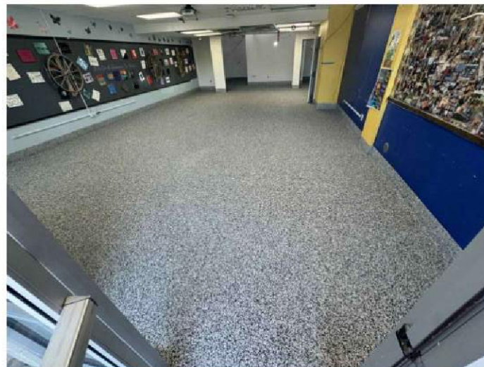
PR08 Epoxy Flooring Complete
