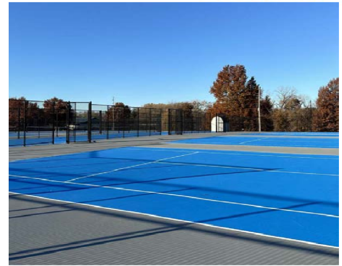
North Courts Looking Southwest
