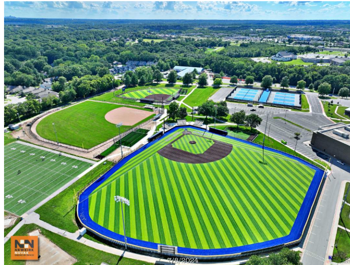
LHS - Overall Site
