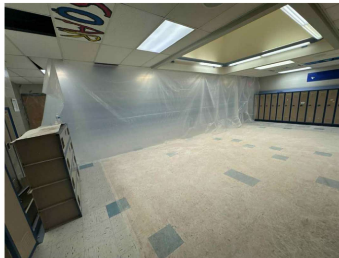
Commons Area (Carpet install in demoed area upcoming)
