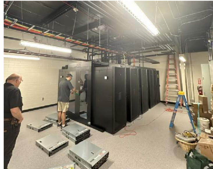
Data Pod Install
