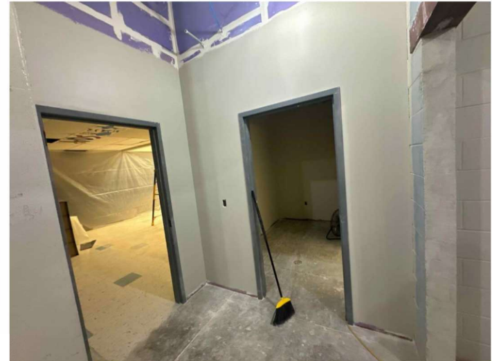
New Door frames for RR/Changing Room
