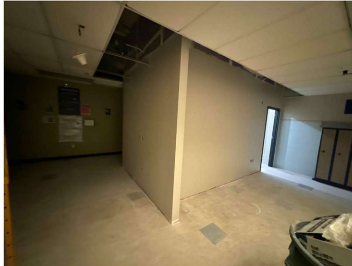
Restroom/Changing room walls
