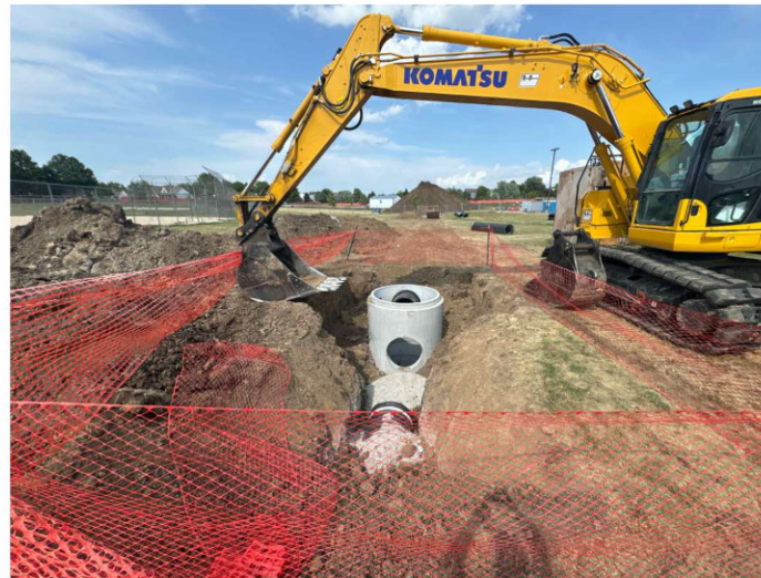
Storm Line Install
