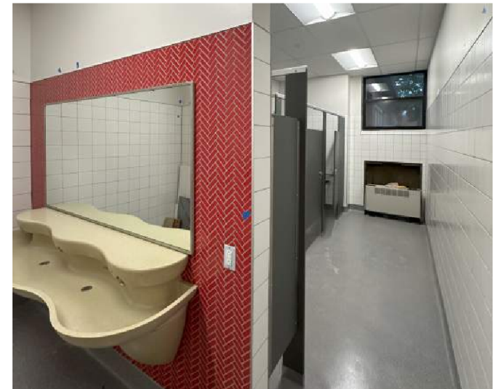
Ridgeview - Level 2 Restroom
