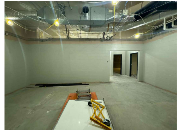
Classroom Prime and Paint
