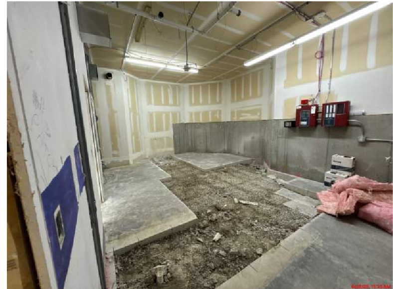
PR08R1 Underground Rough Demo
