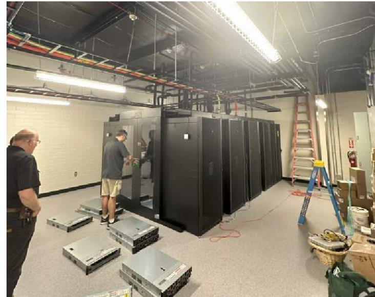
Data Pod Install
