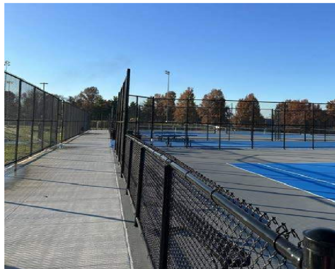
East Concourse Looking South
