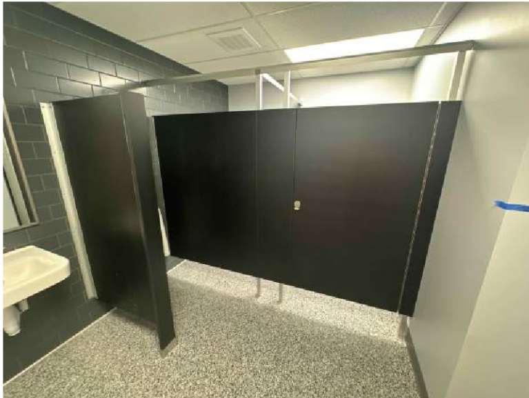
PR03 Men's Restroom (Partitions)
