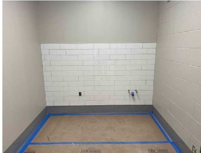
Restroom/Changing room wall tile
