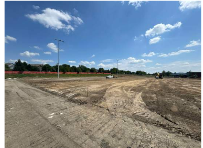
Current Site with new light poles
