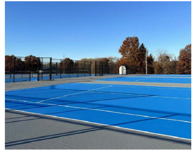
North Courts Looking Southwest
