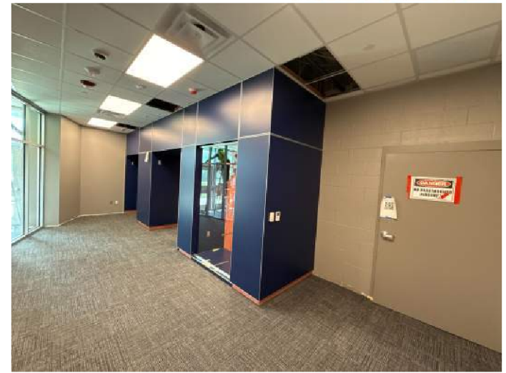
SVMS - Vestibule Wood Laminate Panels
