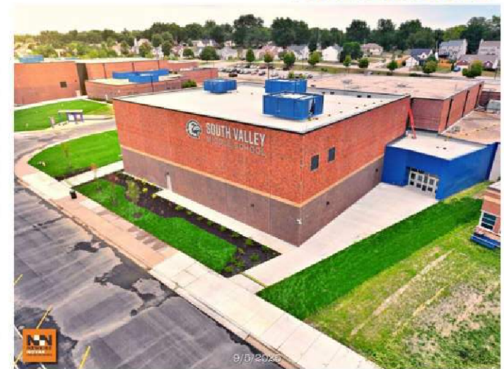
SVMS Exterior View
