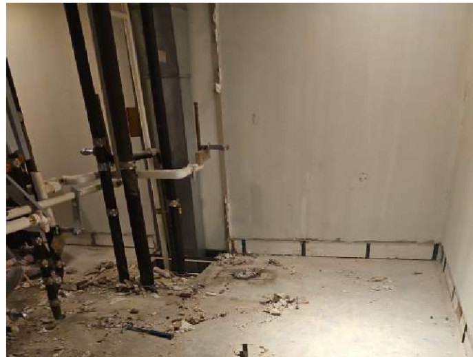
2nd Floor Restrooms
