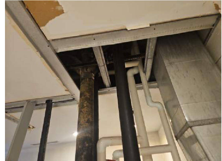
2nd Floor Restrooms
