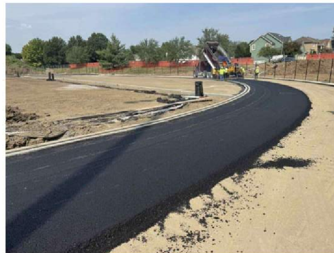
Track Asphalt Base Underway
