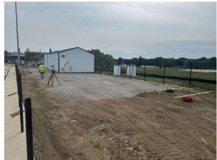
Prepping for Site Concrete
