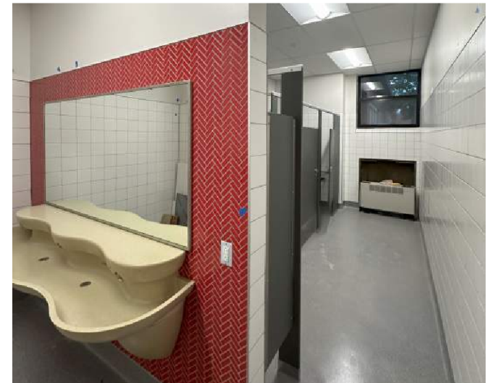
Ridgeview - Level 2 Restroom
