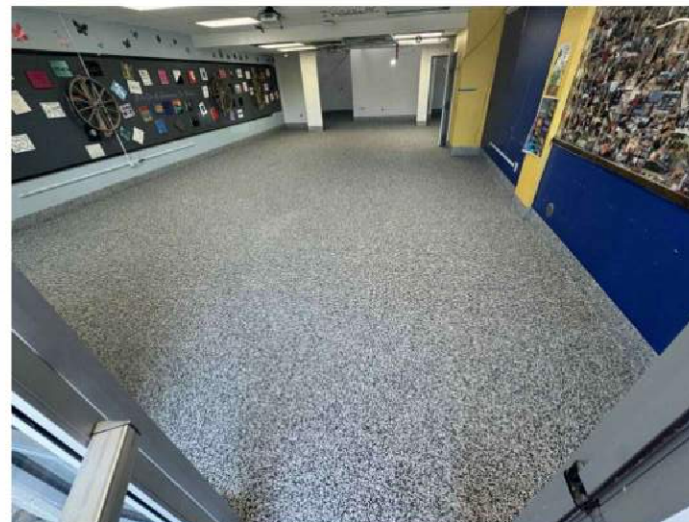
PR08 Epoxy Flooring Complete
