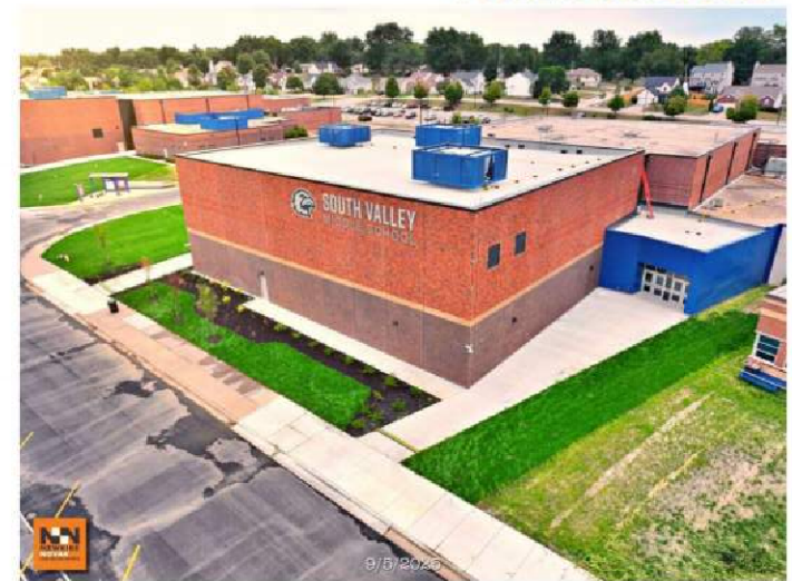
SVMS Exterior View
