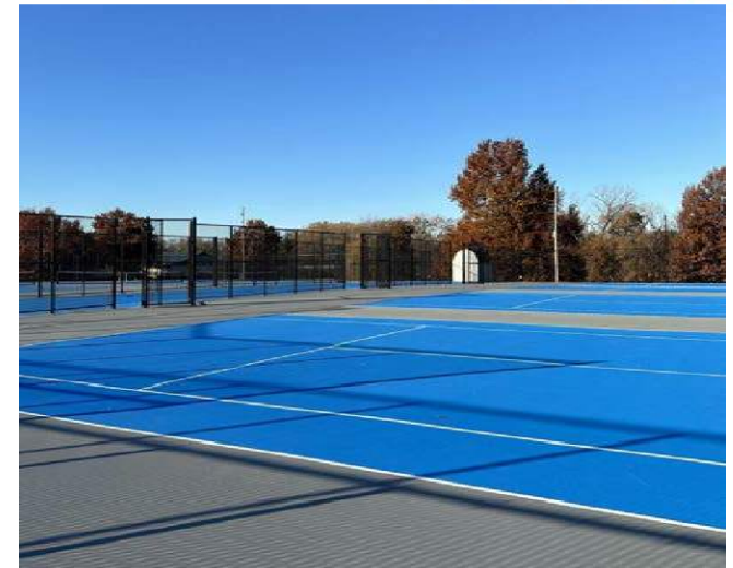
North Courts Looking Southwest
