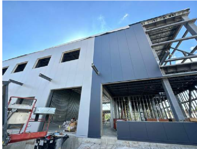
Metal Panels East Wall
