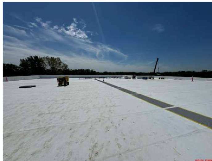
Upper Roofing TPO
