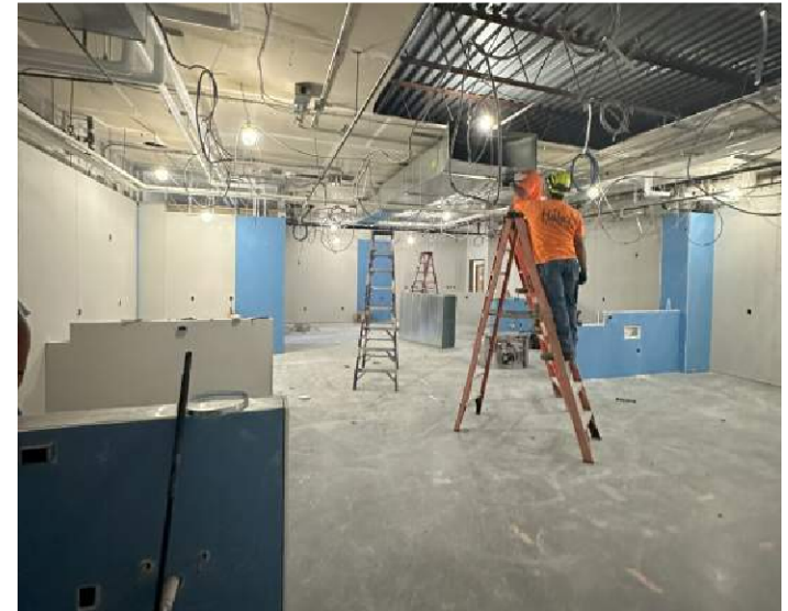
Progress 100's Wing
