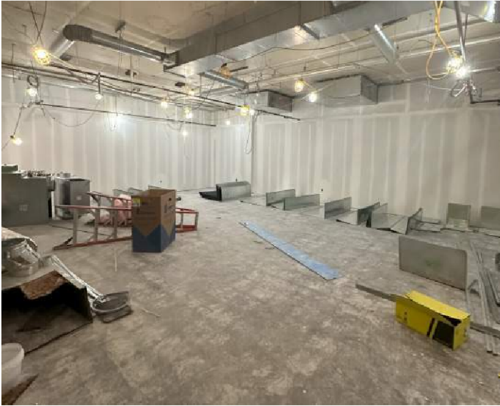
Progress 100's Wing
