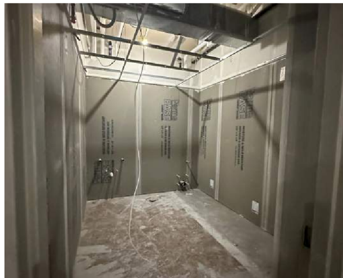
Progress 100's Wing
