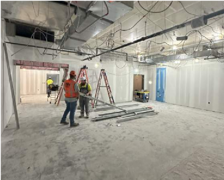
Progress 100's Wing
