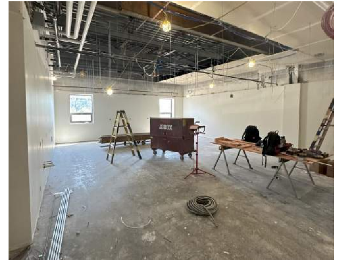
Progress 100's Wing
