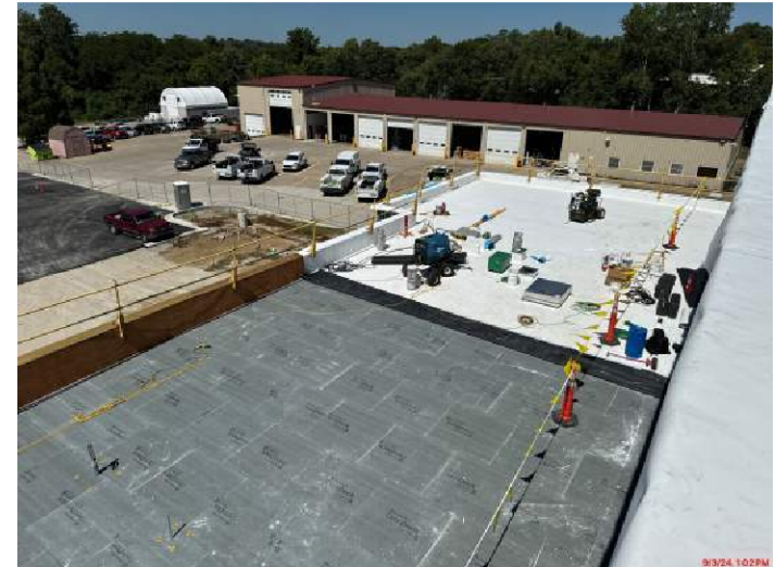
Lower Roofing TPO
