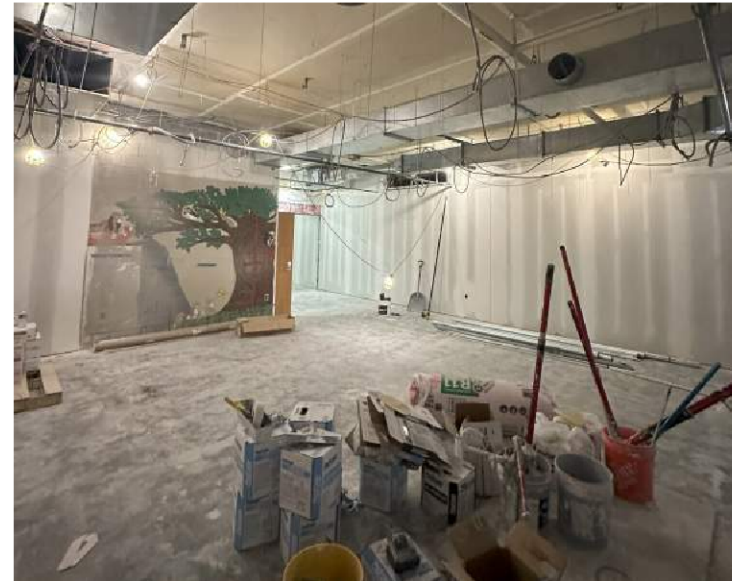
Progress 100's Wing
