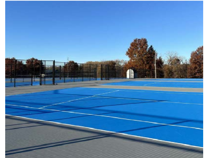
North Courts Looking Southwest
