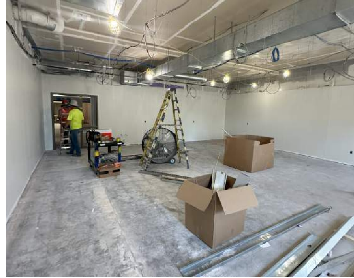
Progress 100's Wing
