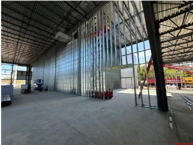
Warehouse Divider Wall
