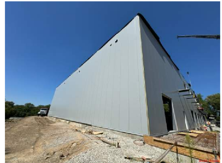
Metal Panels South Wall
