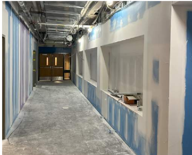
Progress 100's Wing
