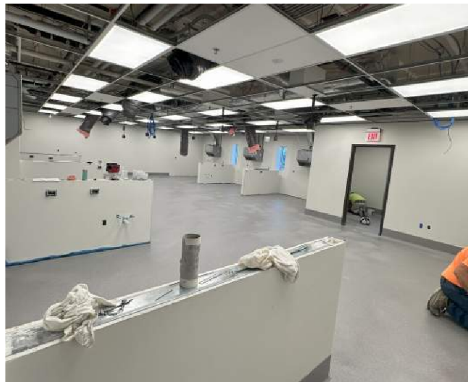
Progress 100's Wing
