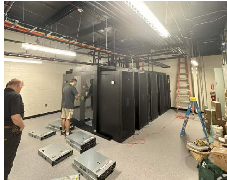
Data Pod Install
