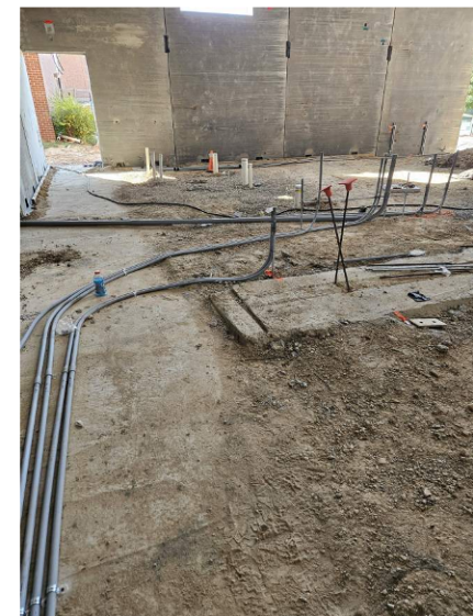
DMS - MEP Under-slab
