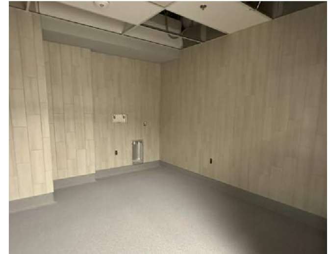
Progress 100's Wing
