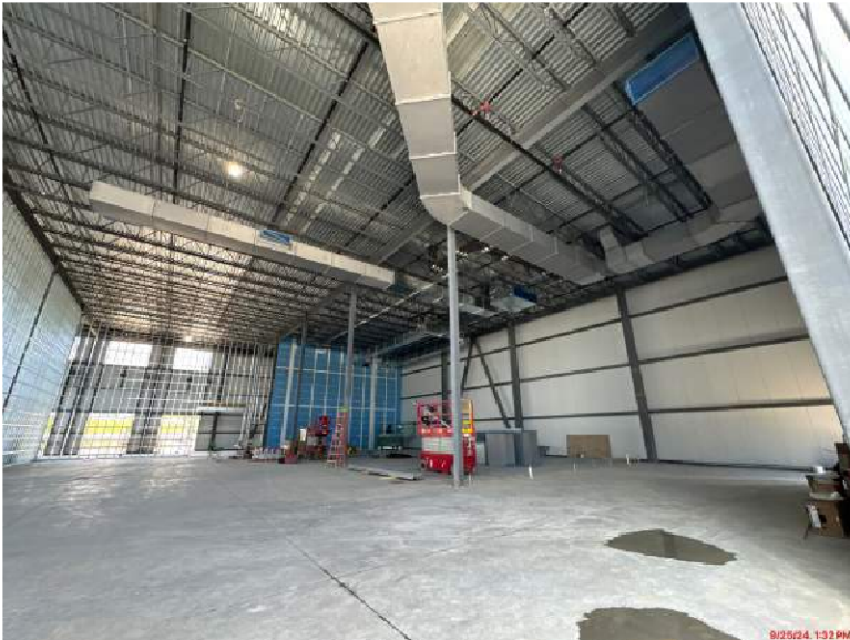
Dry Storage / Freezer
