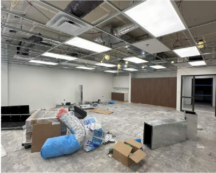
Progress 100's Wing
