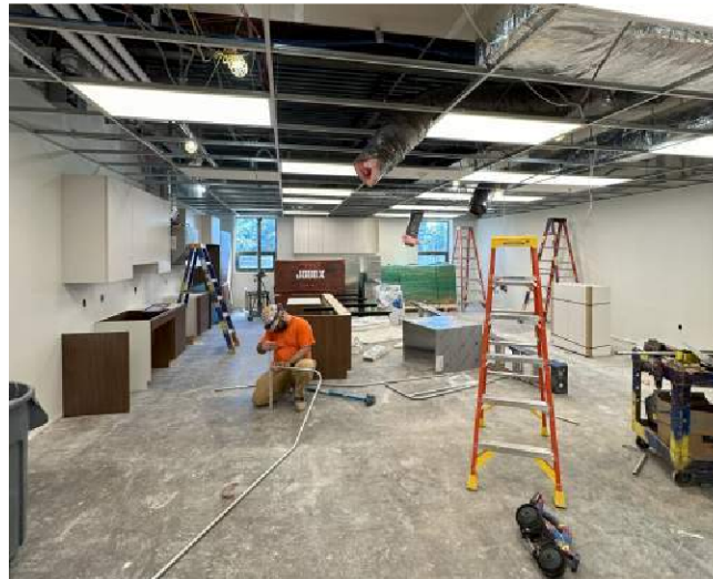
Progress 100's Wing
