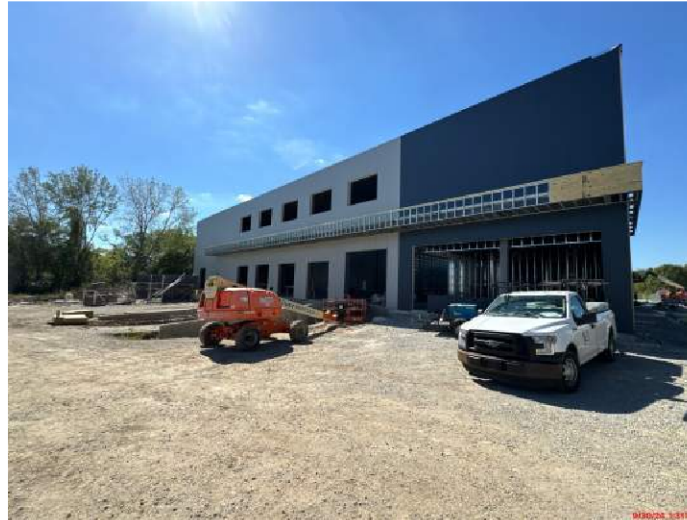
Metal Panels East Wall
