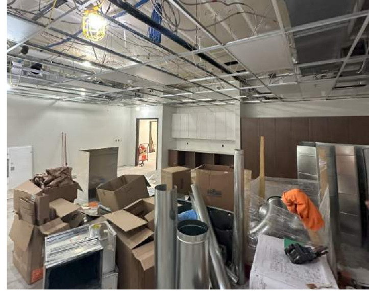
Progress 100's Wing
