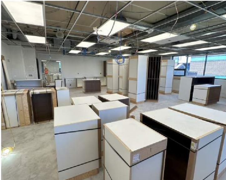
Progress 100's Wing
