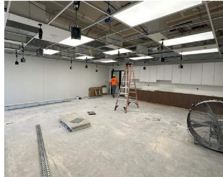
Progress 100's Wing
