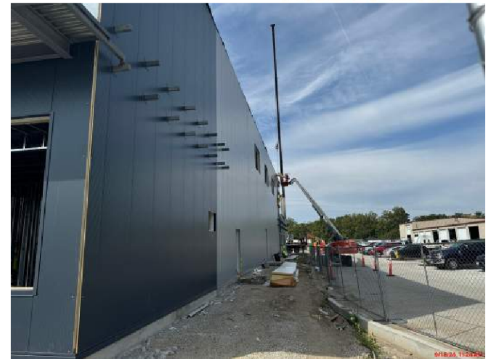
Metal Panels North Wall
