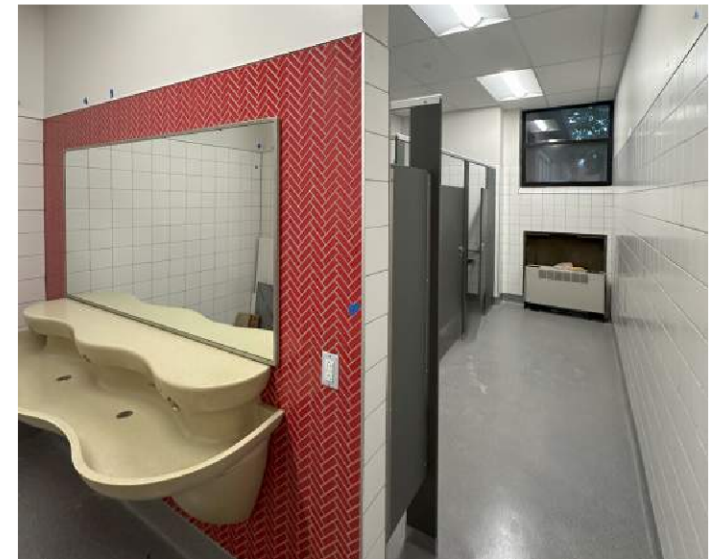
Ridgeview - Level 2 Restroom
