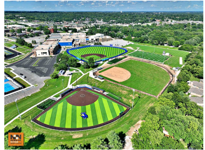
LHS - Overall Site
