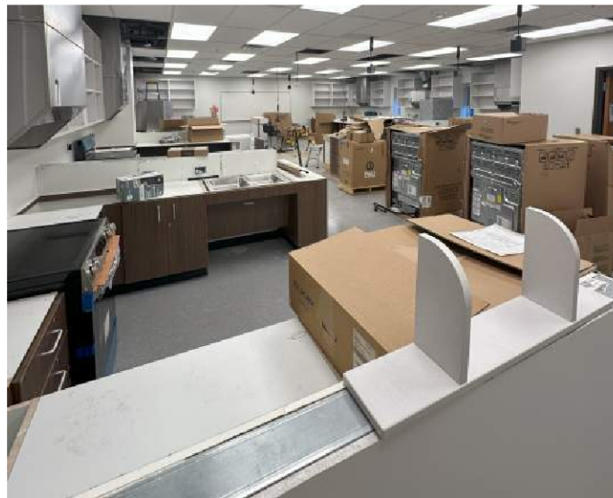
Progress 100's Wing
