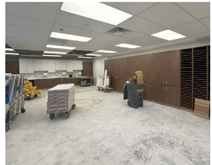
Progress 100's Wing
