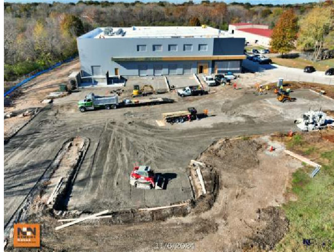
East Lot Construction
