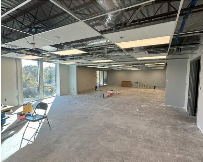
1964 (Area A) Progress
