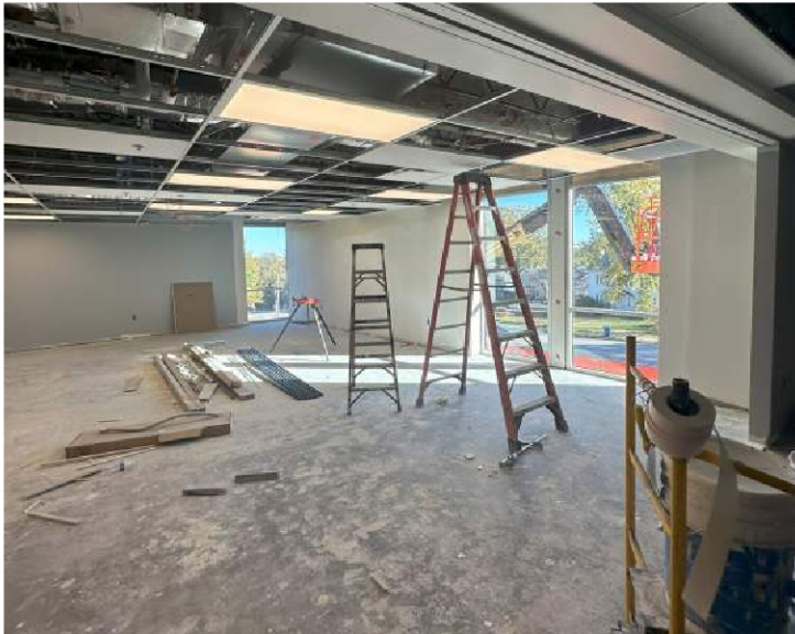
1964 (Area A) Progress
