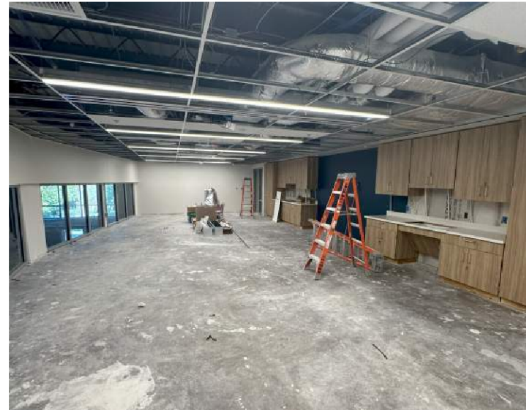
1964 (Area A) Progress
