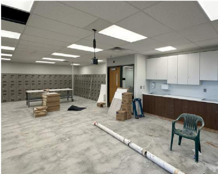
Progress 100's Wing
