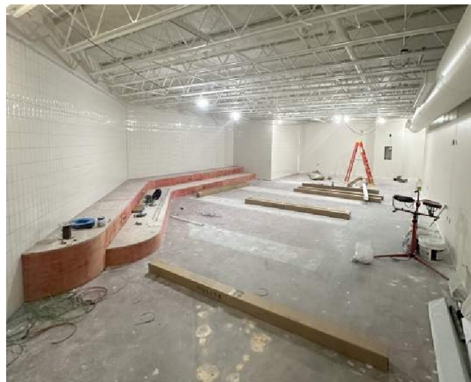
1964 (Area A) Progress
