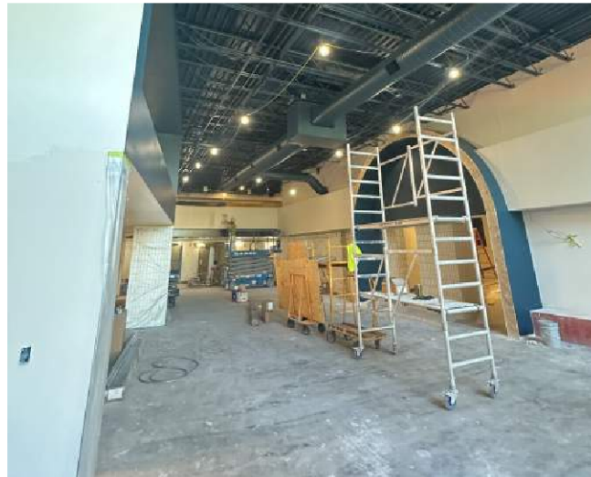
1964 (Area A) Progress
