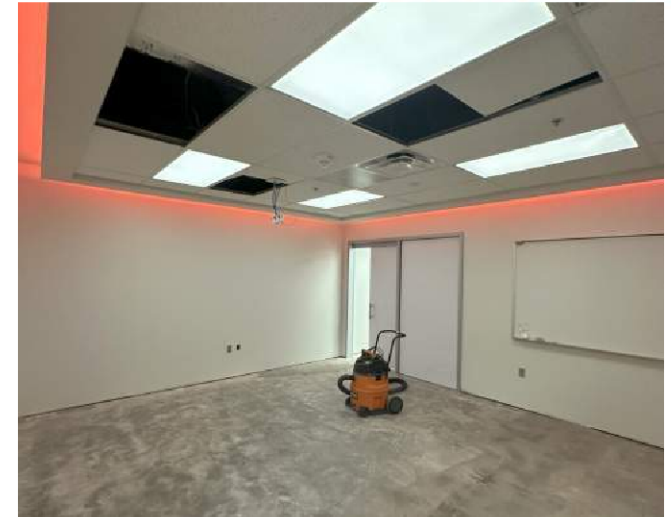
Progress 100's Wing
