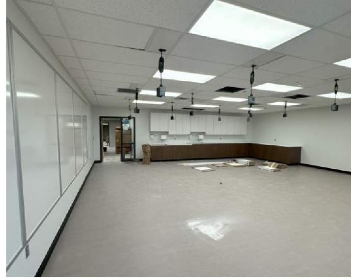
Progress 100's Wing
