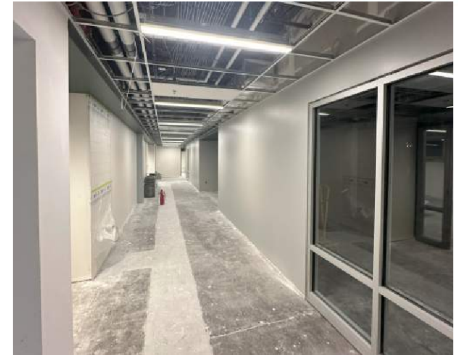
1964 (Area A) Progress
