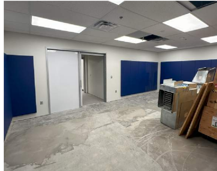
Progress 100's Wing
