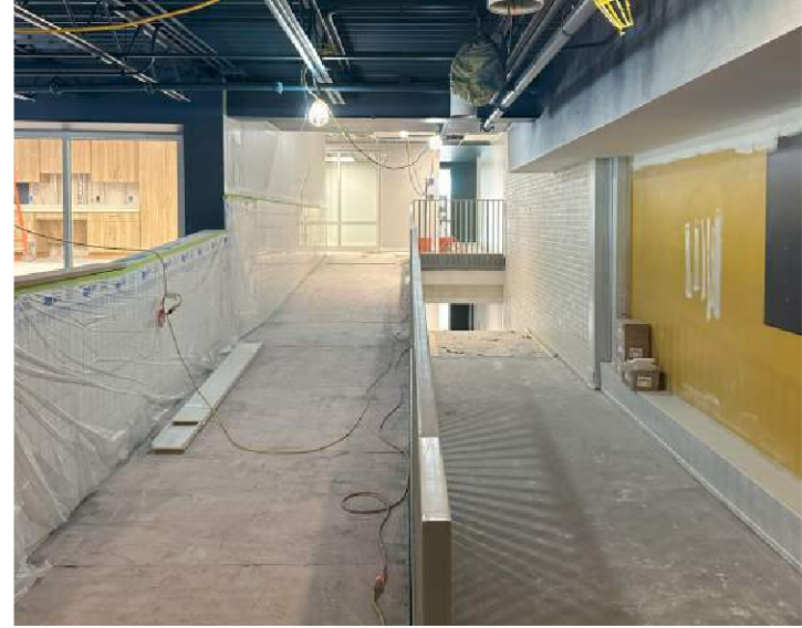
1964 (Area A) Progress
