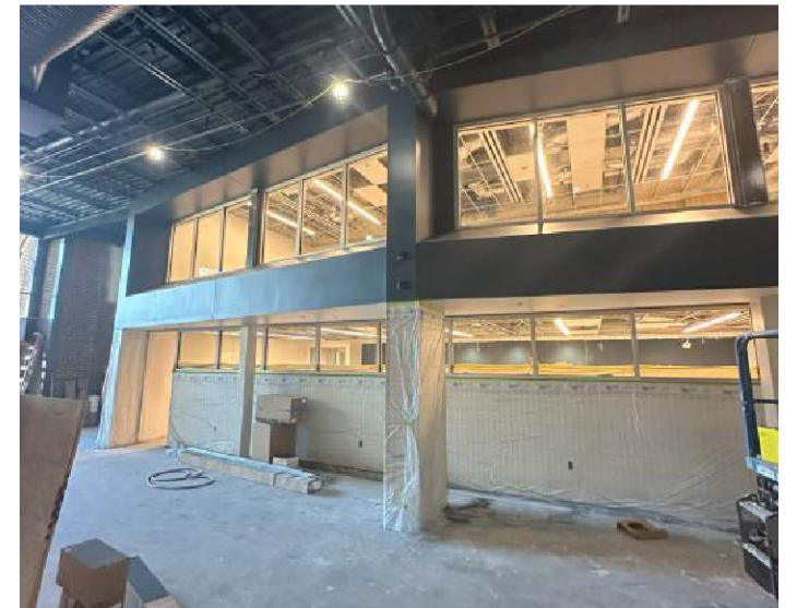
1964 (Area A) Progress
