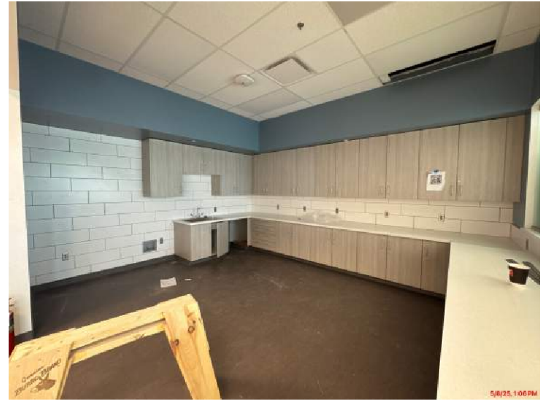
Break Room A103
