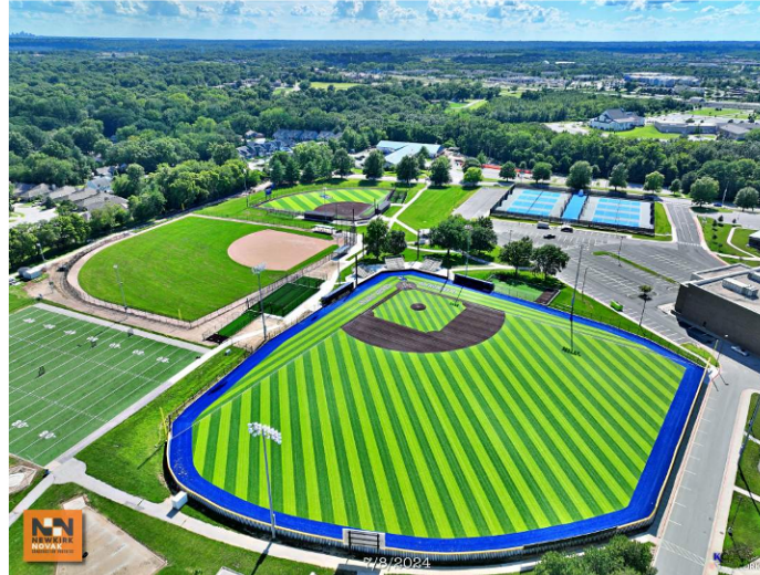
LHS - Overall Site
