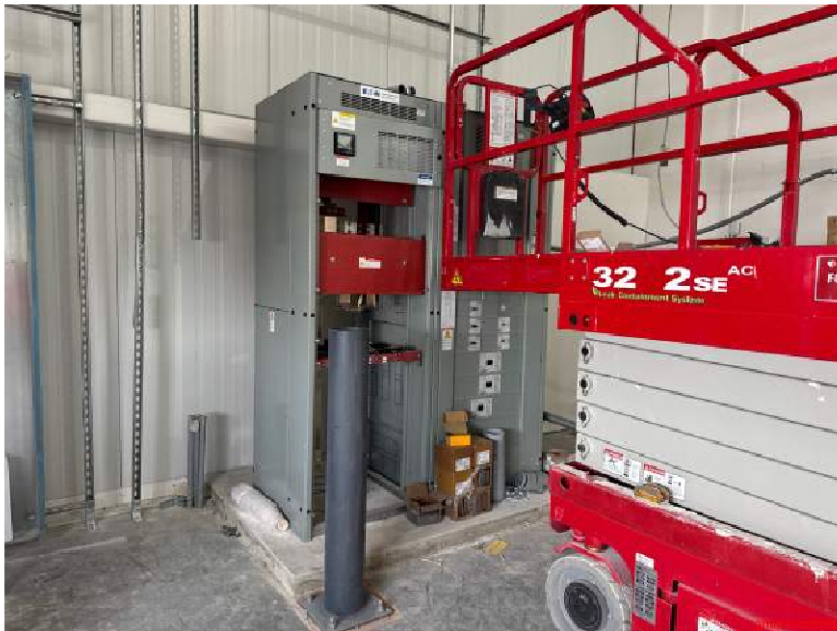
Distribution Gear Install
