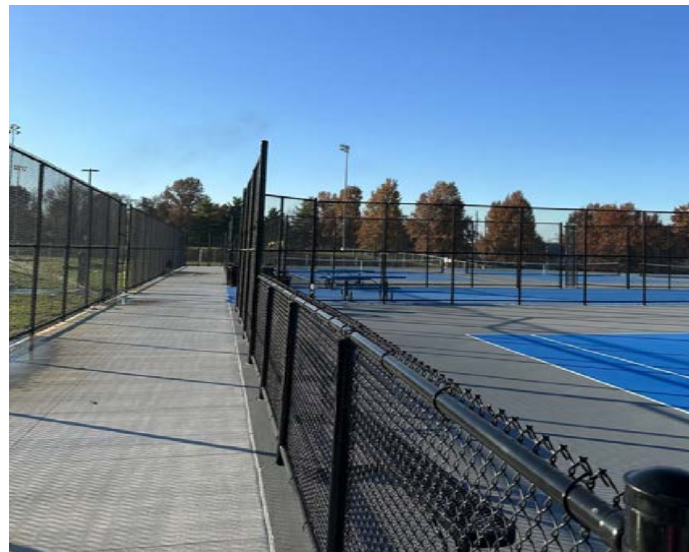
East Concourse Looking South
