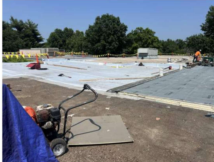
Alexander Doniphan - Roof Replacement
