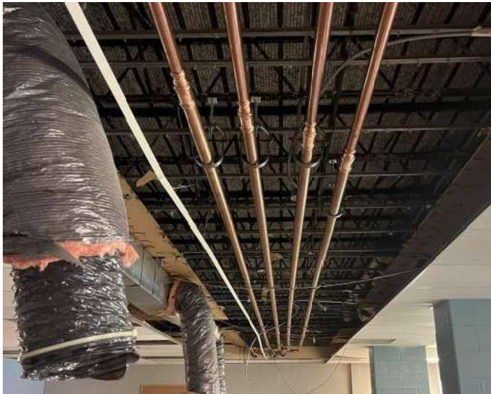
Ridgeview - New Mechanical Piping Install
