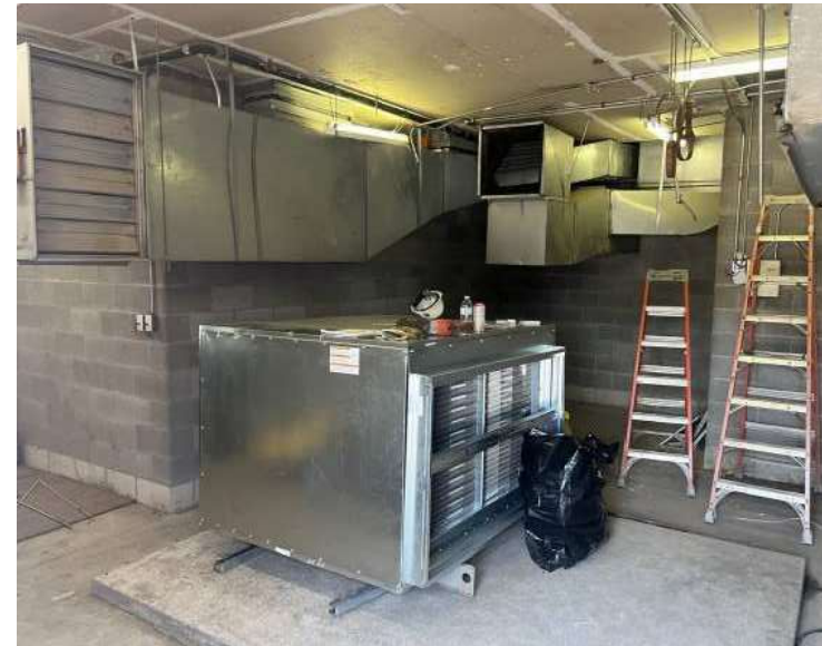
Ridgeview - New HVAC Unit Install
