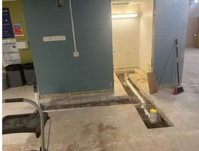
Under slab rough in
