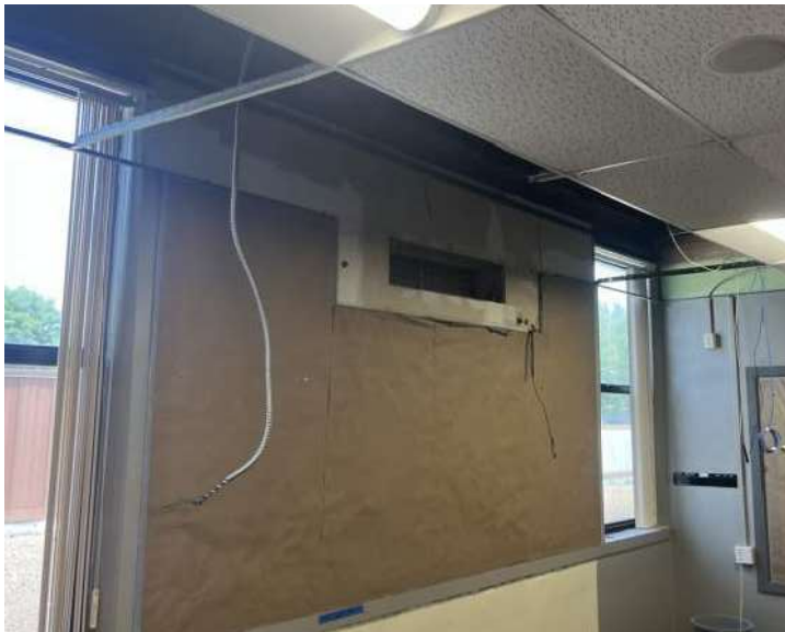
Ridgeview - Existing HVAC Unit Removal
