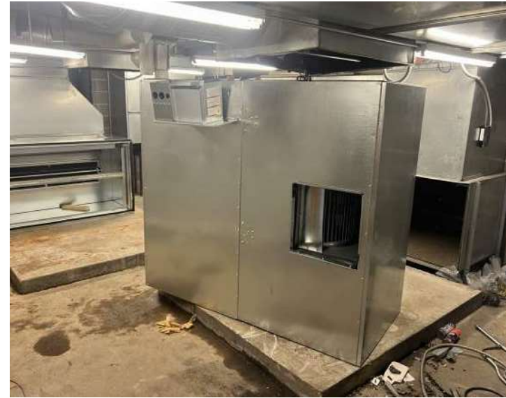
Ridgeview - New HVAC Unit Install
