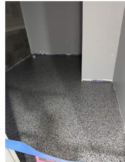
Epoxy flooring PR03
