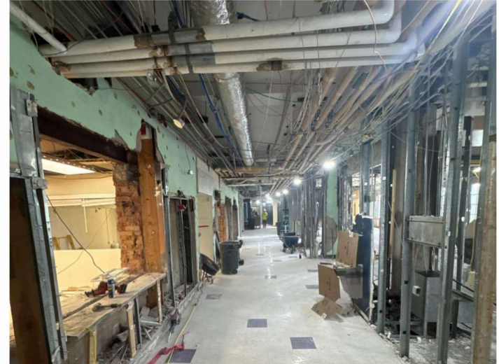
1st Floor Corridor
