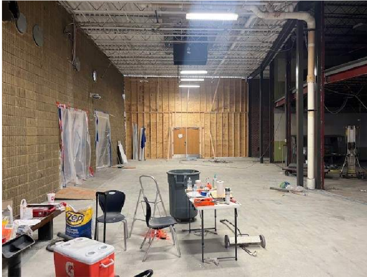
1964 (Area A) Progress
