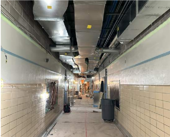
Ridgeview - Corridor MEP Install
