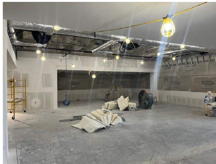
New Seating Area Progress
