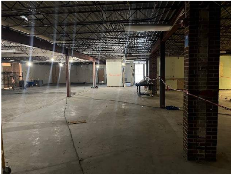
1964 (Area A) Progress
