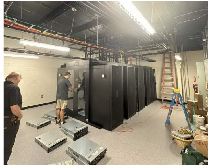
Data Pod Install
