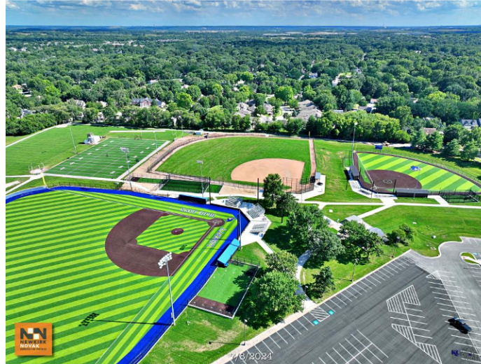
LHS - Overall Site
