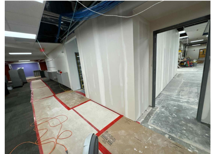
EPiC Elementary - Interior Renovation
