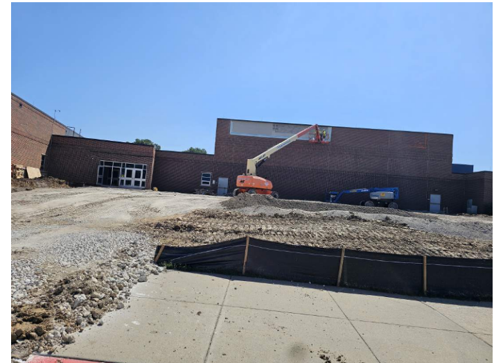
DMS - Building Pad
