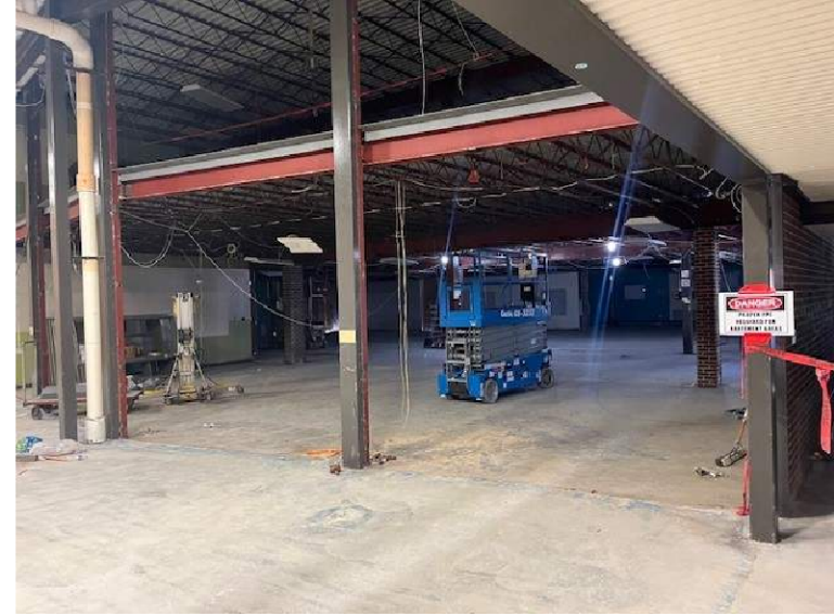
1964 (Area A) Progress
