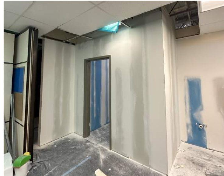
Doniphan - SPED Restroom Remodel
