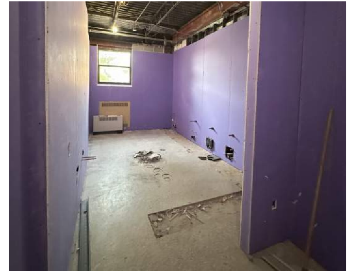
Ridgeview - Level 2 Restroom
