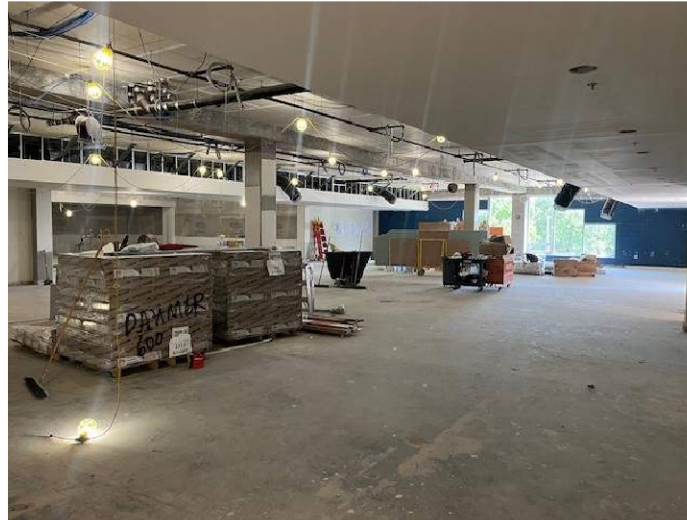
Cafeteria Build Back
