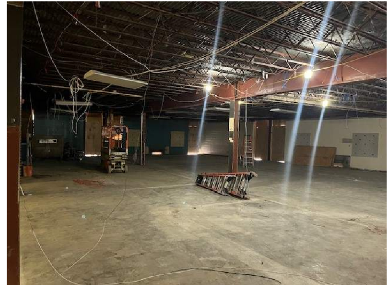
1964 (Area A) Progress
