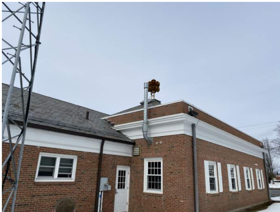
● D2. 6: Community Alert Siren Mounted on Roof
