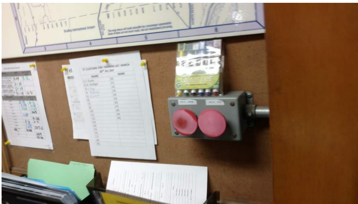
● D2. 43: Traffic Signal Control Buttons (1)
