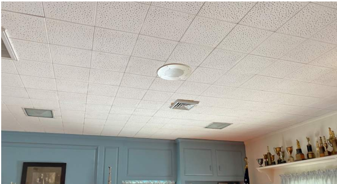
● D2. 10: Diffuser in Ceiling Served by Fan Coil Unit
