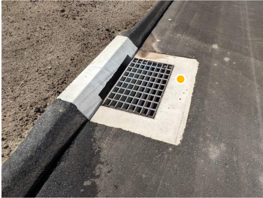
● D3. 5: New catch basins and tops were recently installed
