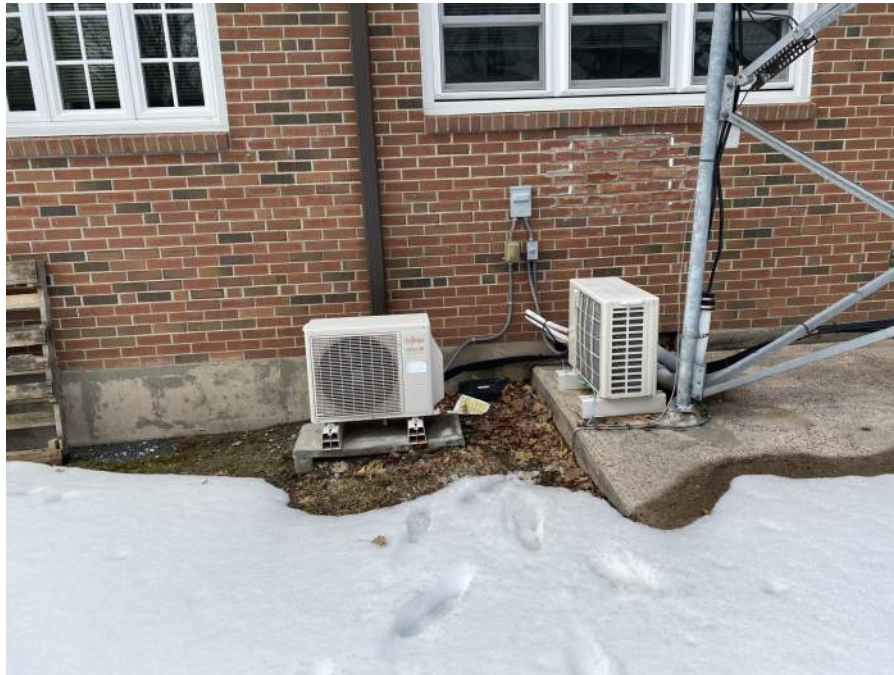
● D2. 9: Condensing Units Serving IT Room Split Units Providing Cooling
