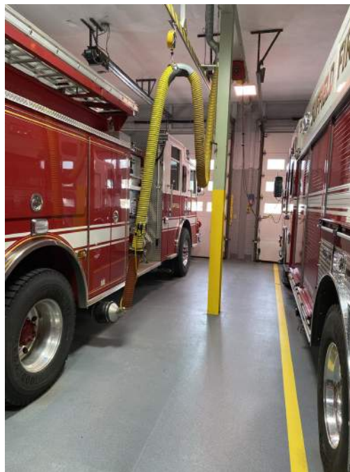
● D2. 36: Plymovent Exhaust
