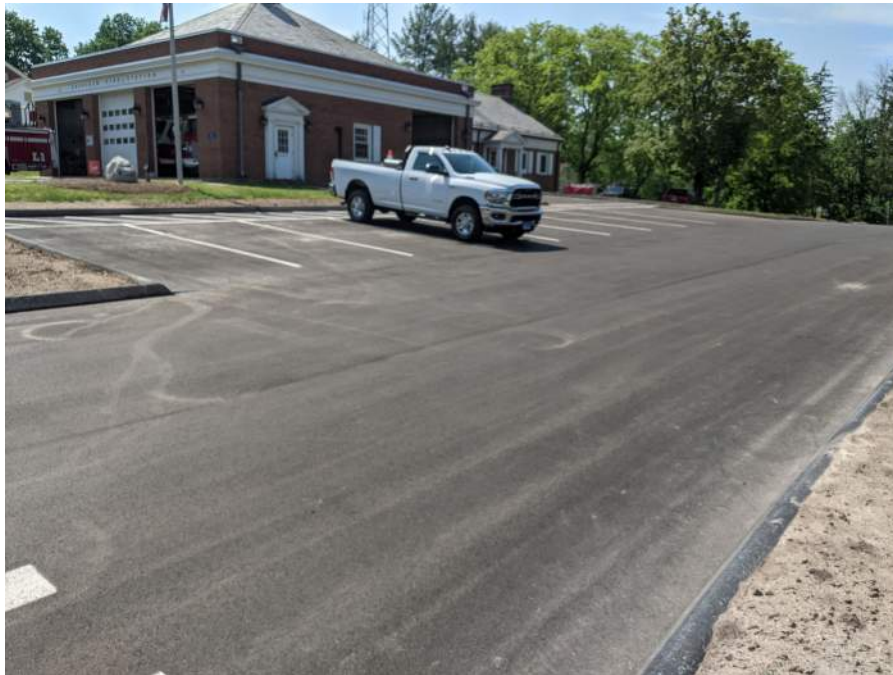
● D3. 1: Parking area and drive aisle West of the building has been recently replaced
