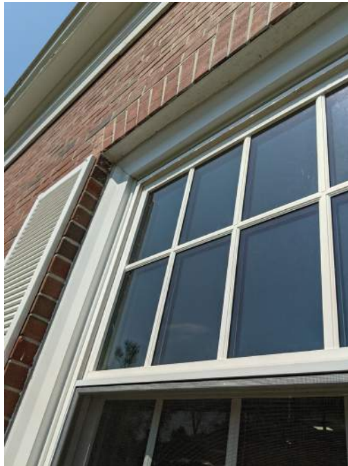
● D1. 9: Aluminum windows located throughout
