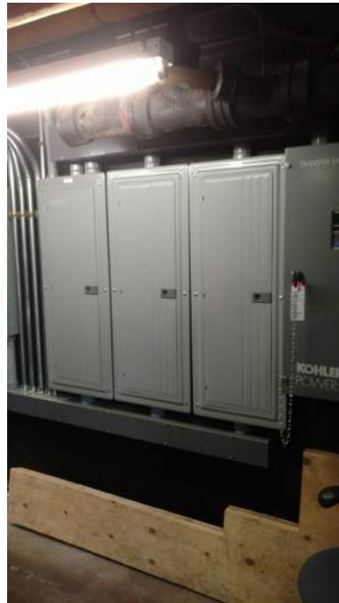
● D2. 5: Branch Circuit Panelboards
