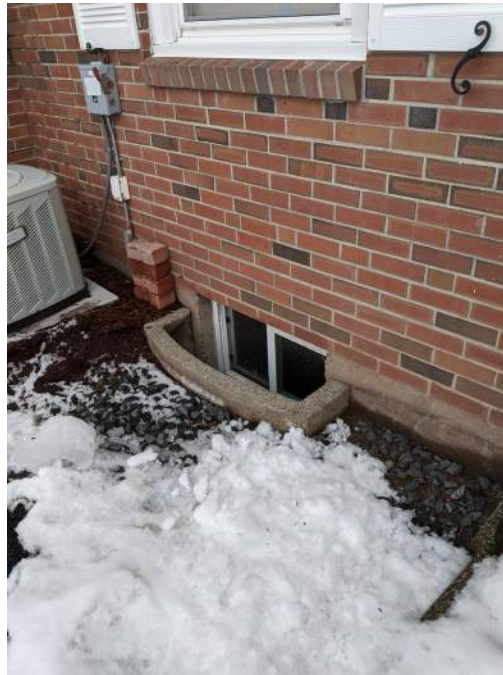
● D1. 3: Window well to lower level
