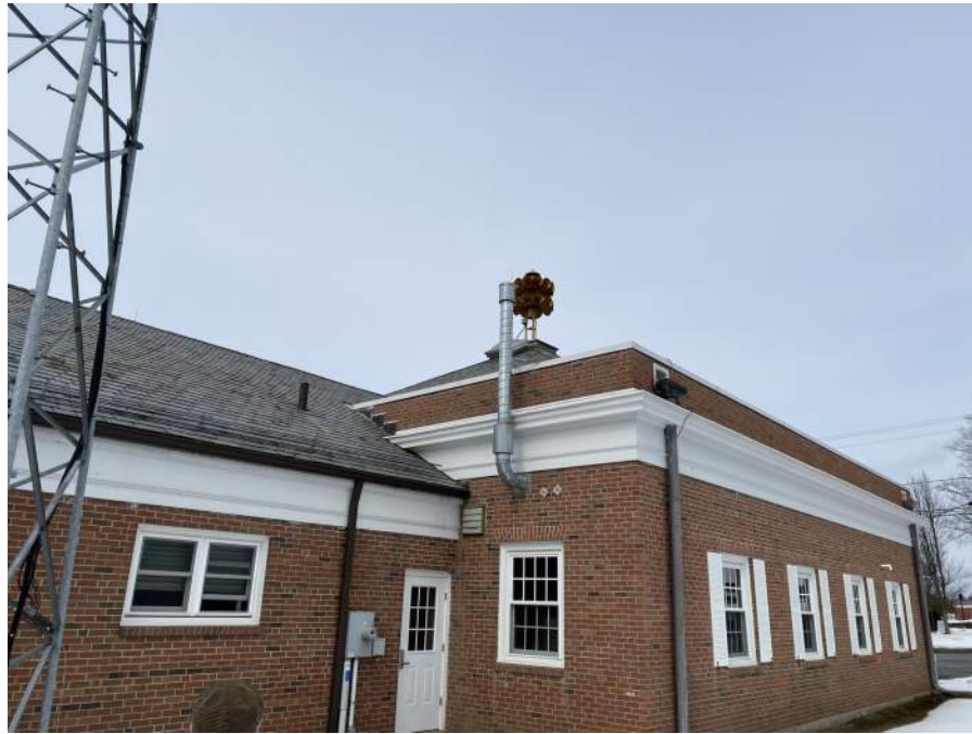
● D2. 39: Roof Drain Gutters and App Bay Exhaust
