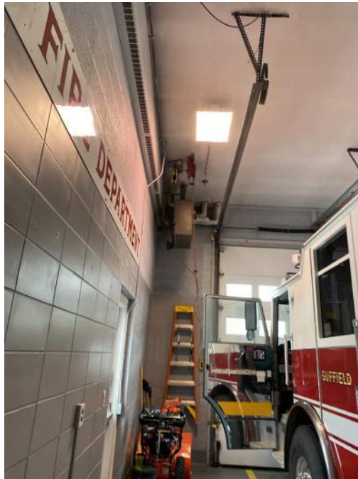
● D2. 17: Hot Water Unit Heater in App Bay
