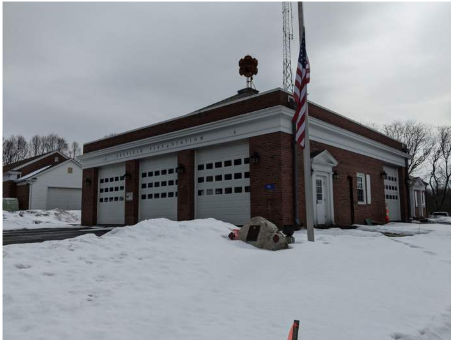
● D1. 1: Northwest corner
