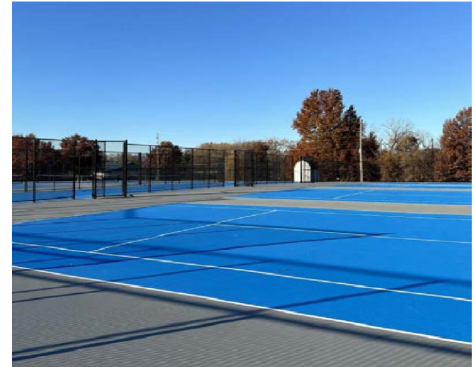
North Courts Looking Southwest
