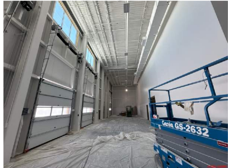
Garage Doors/Ceiling Paint
