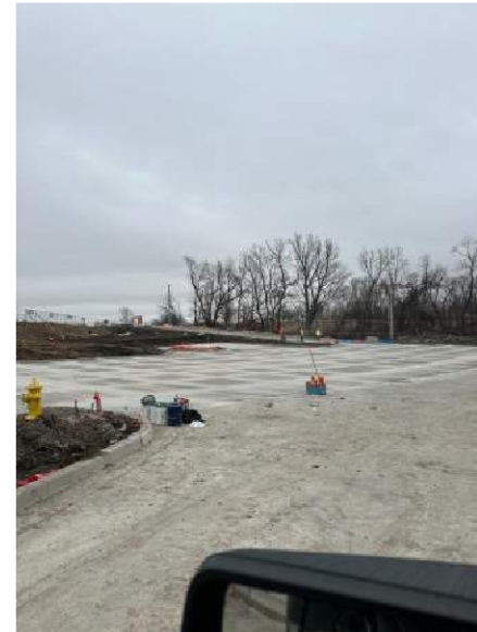
East Lot paving
