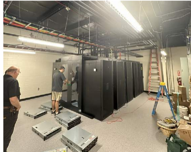
Data Pod Install
