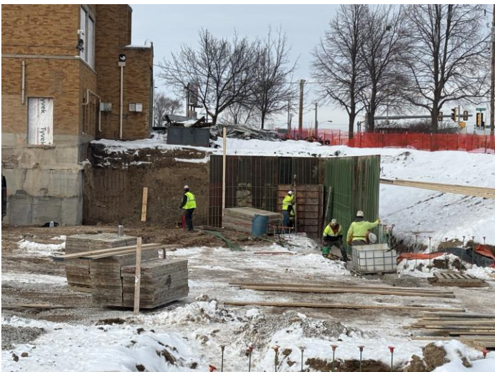
Foundation walls eastside of building B
