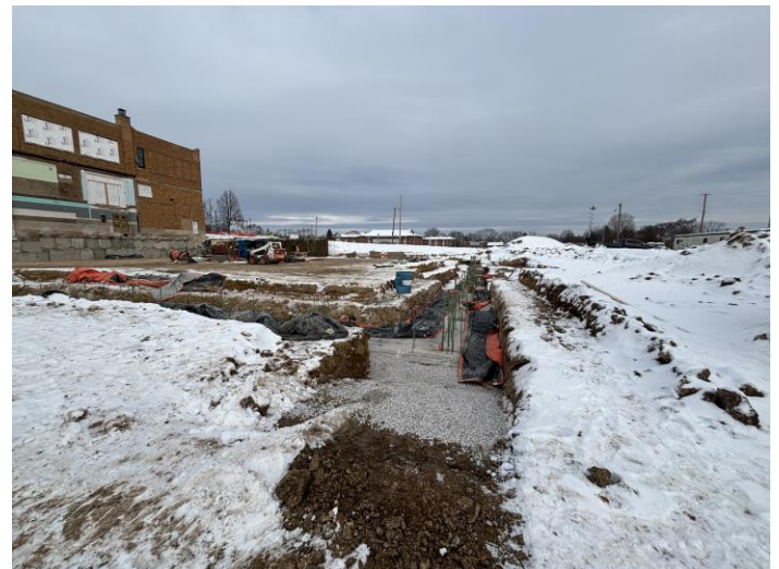
Footings on southwest corner of building B
