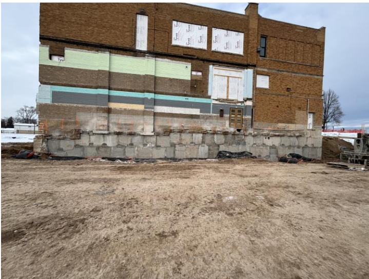
Underpinning building A south elevation.
