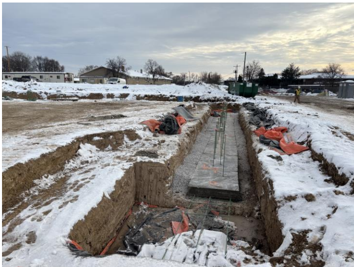
Footings on west side building B
