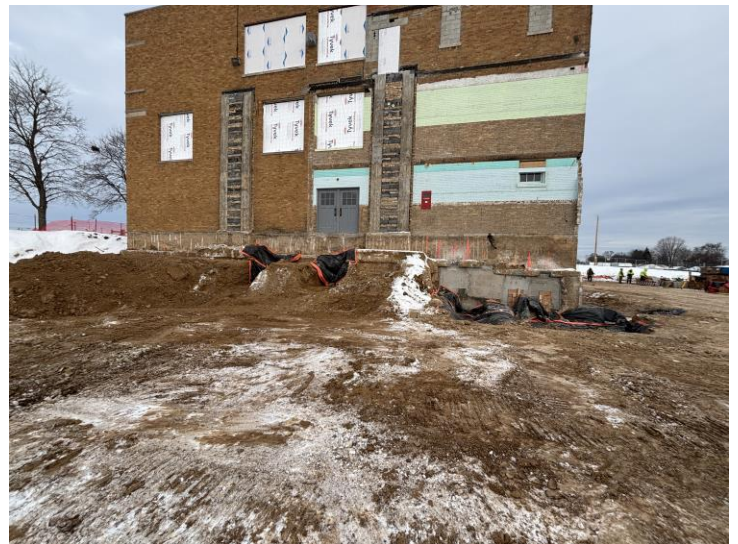
Underpinning building A west elevation
