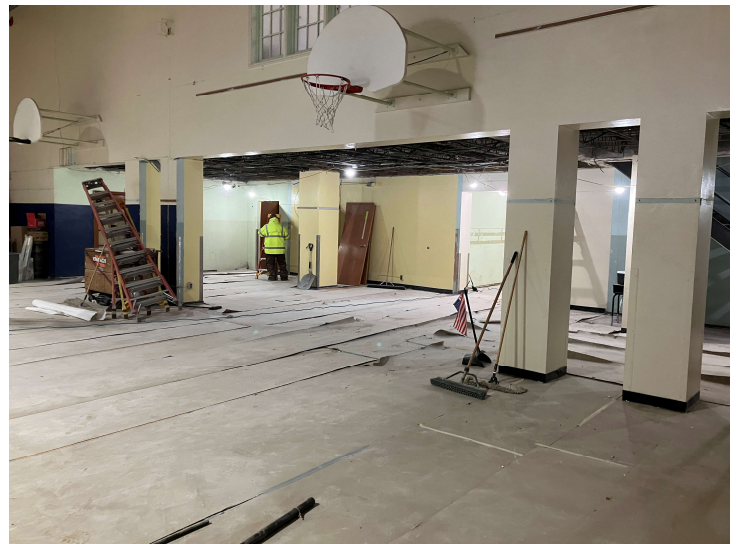
First floor Selective demolition
