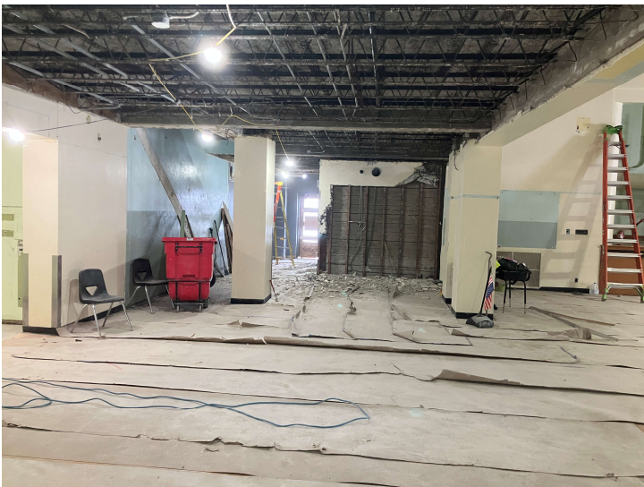
First floor Selective demolition
