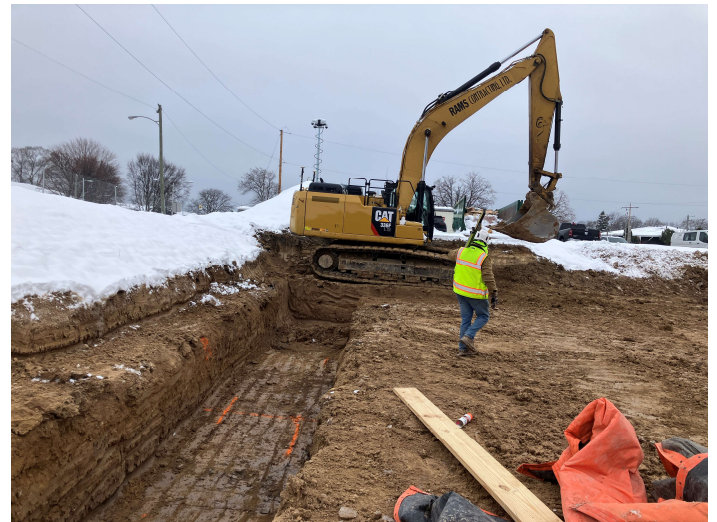
Footings on south end of building A
