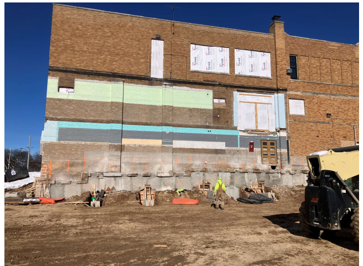
Underpinning south of building A
