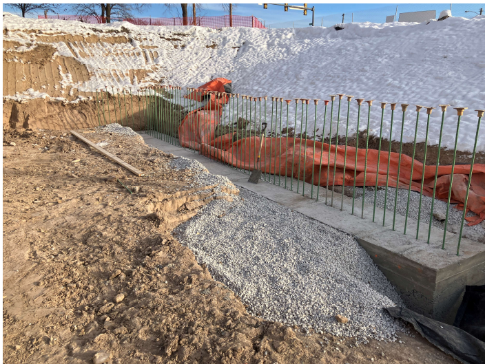
Footings on south end of building A
