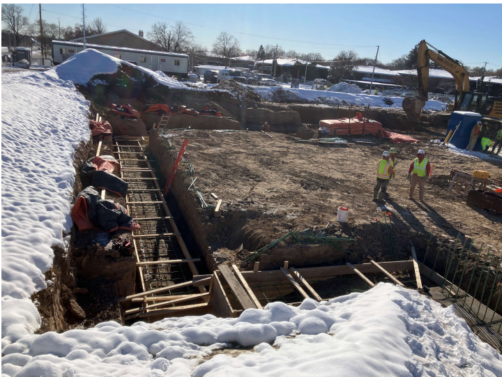
Underpinning south end of building A
