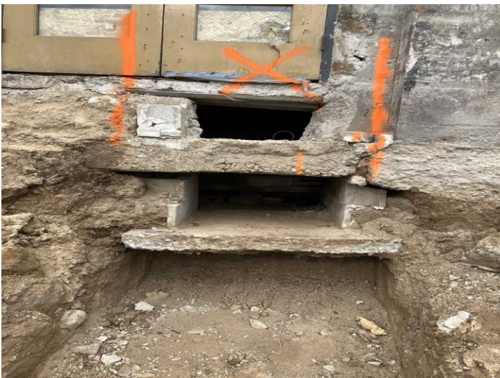
Underpinning south end of building area A
