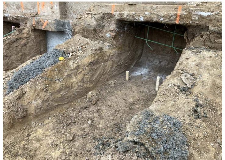
Underpinning South side of area A
