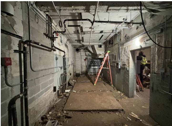
Boiler room demolition
