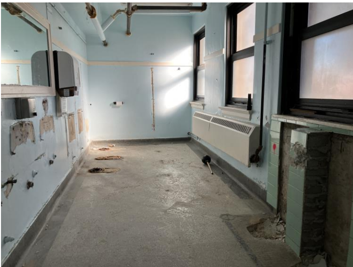
Bathroom selective demolition
