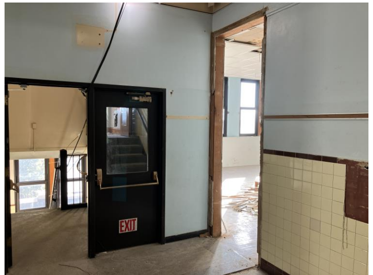
Interior selective demolition
