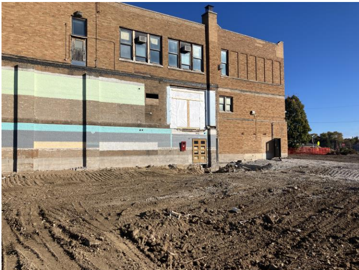
Temporary enclosure installed at building connection
