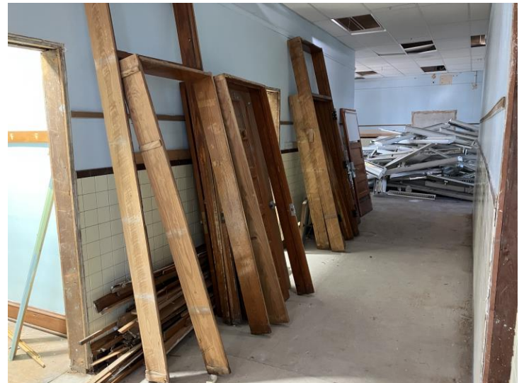
Salvaging wood doors & frames
