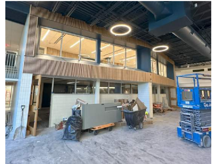
1964 (Area A) Progress
