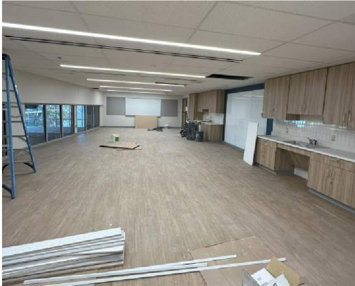
1964 (Area A) Progress
