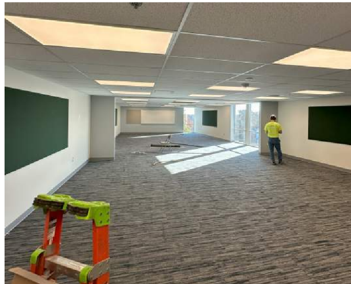
1964 (Area A) Progress
