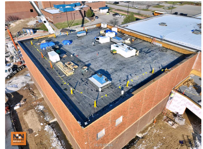
SVMS - Gym Roofing
