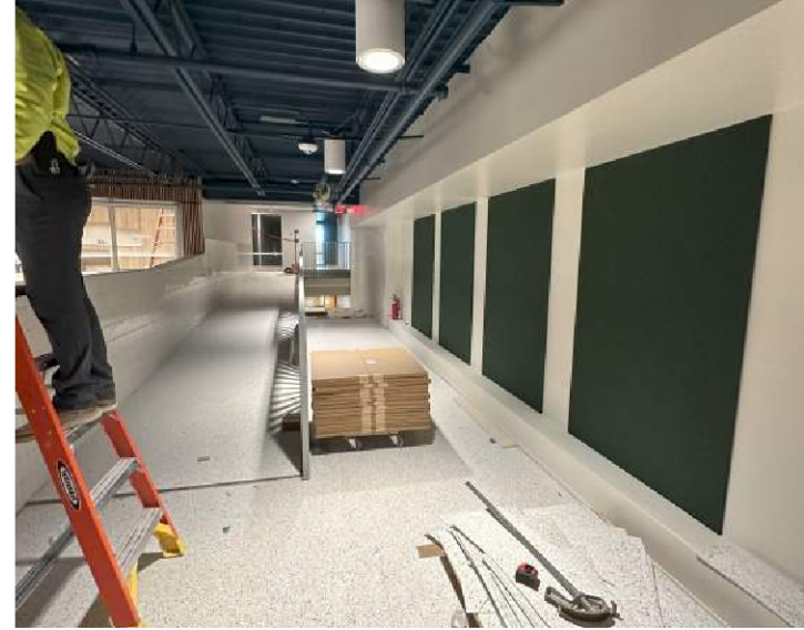
1964 (Area A) Progress
