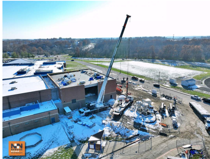
SVMS - Pre-cast panel leave out install
