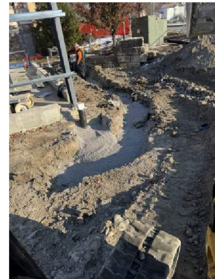
PR04 Storm Drains
