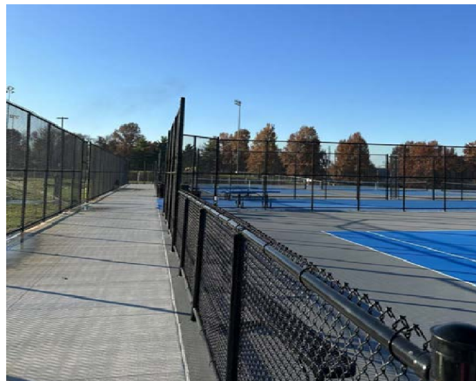
East Concourse Looking South
