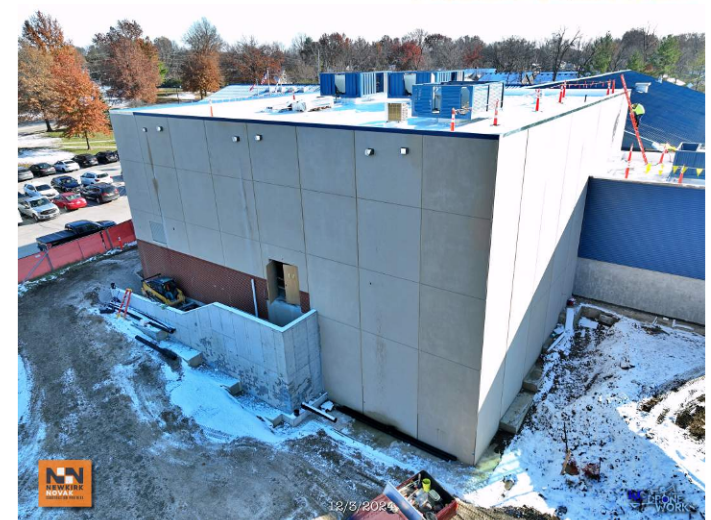
EPiC Elementary - N. Retaining Wall
