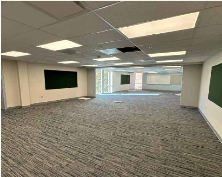
1964 (Area A) Progress
