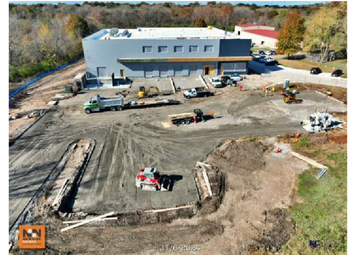
East Lot Construction
