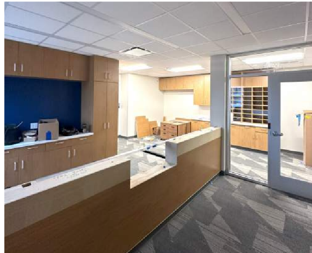
Franklin - Main Office
