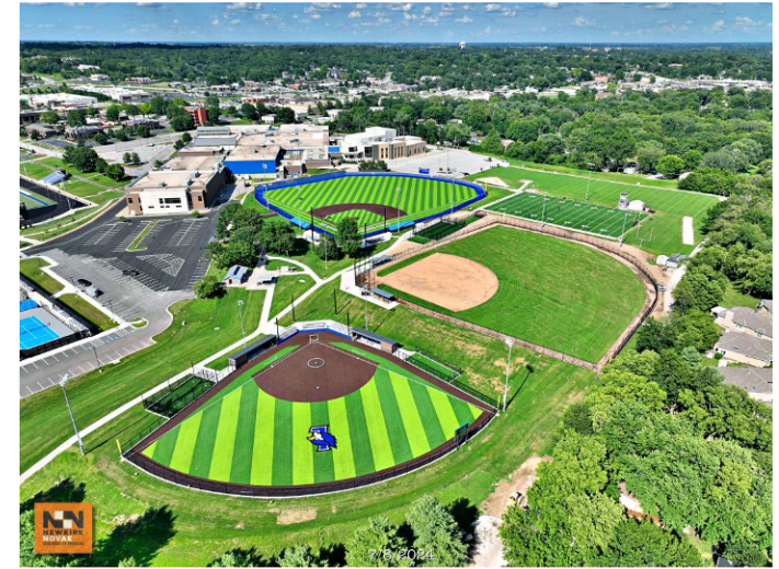
LHS - Overall Site
