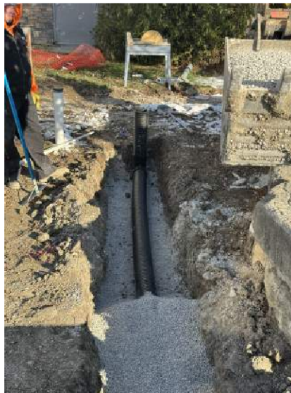
PR04 Storm Drains
