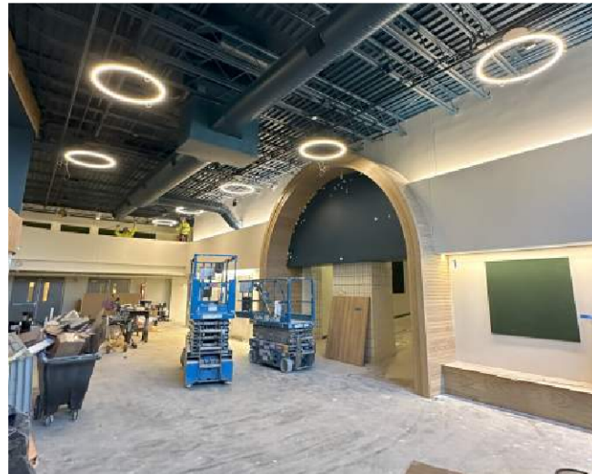
1964 (Area A) Progress
