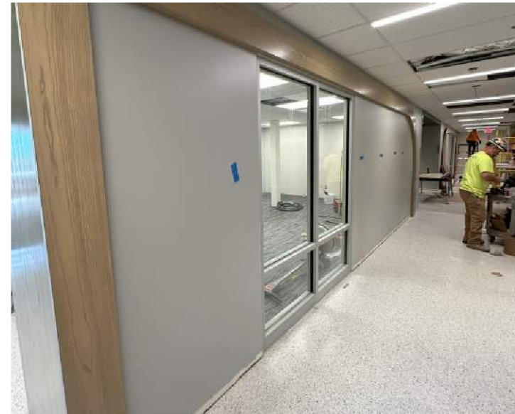
1964 (Area A) Progress
