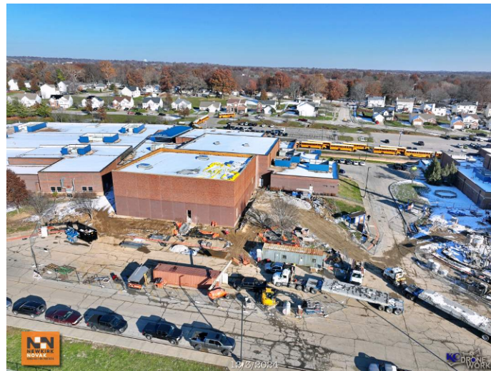
DMS - Pre-cast leave out panels installed
