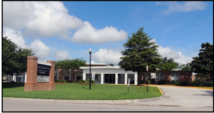
Existing Site of Goodwin Elementary School
