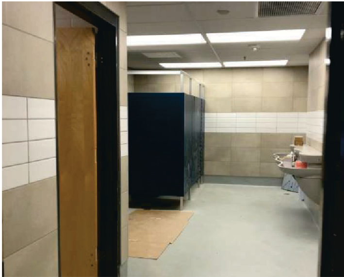
Restroom Build Back
