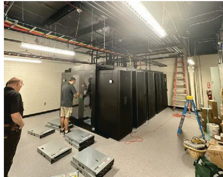
Data Pod Install
