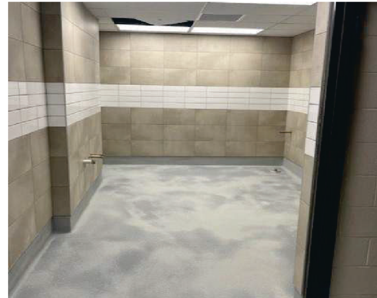
Restroom Build Back
