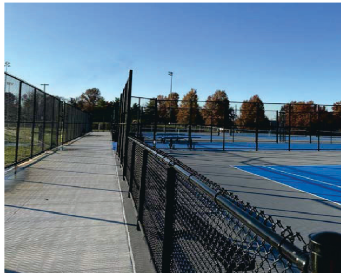
East Concourse Looking South
