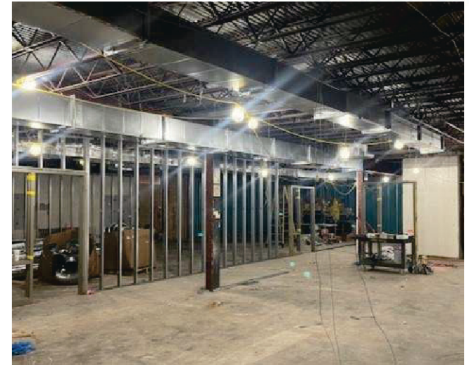
1964 (Area A) Progress
