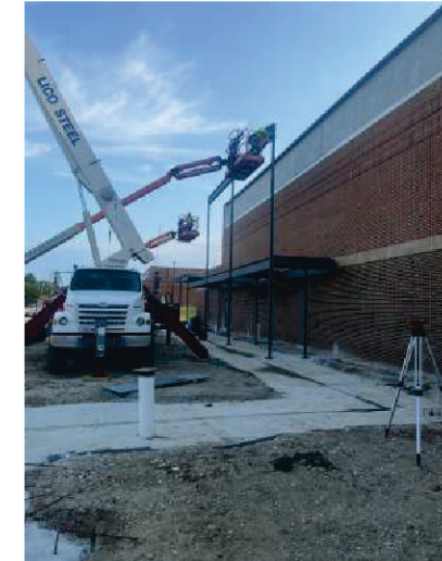
SVMS - Steel Erection
