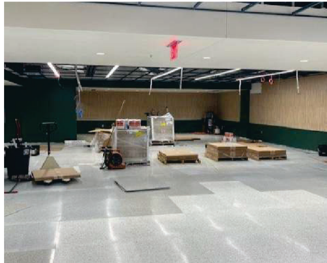
Cafeteria Build Back
