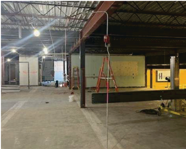
1964 (Area A) Progress
