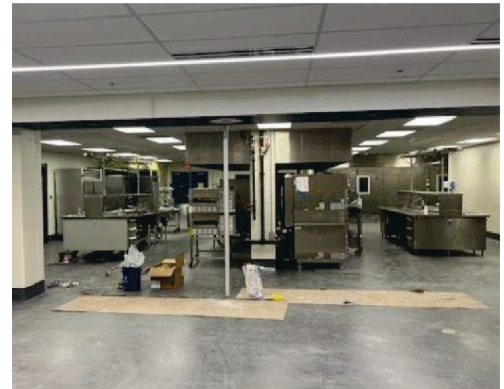
Kitchen Build Back
