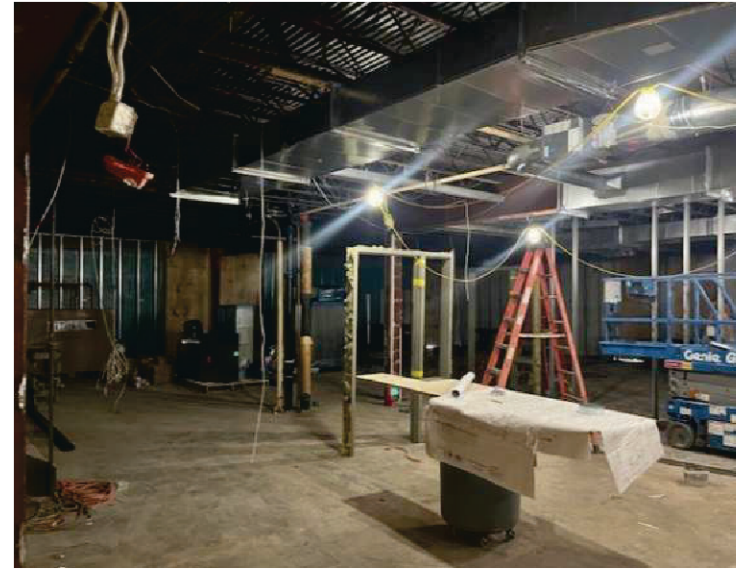
1964 (Area A) Progress
