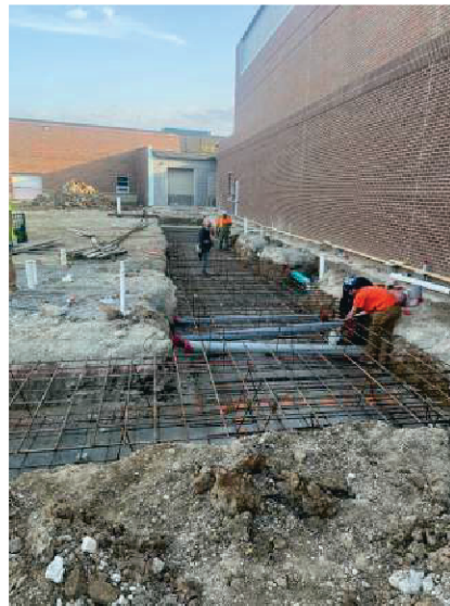
DMS - Footing Rebar
