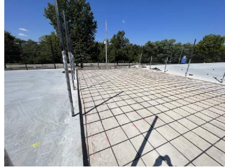
Center Spectator Area Slab Prep / Reinforcing
