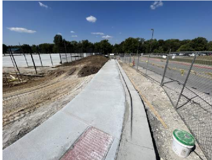
Looking West Curb and Sidewalk
