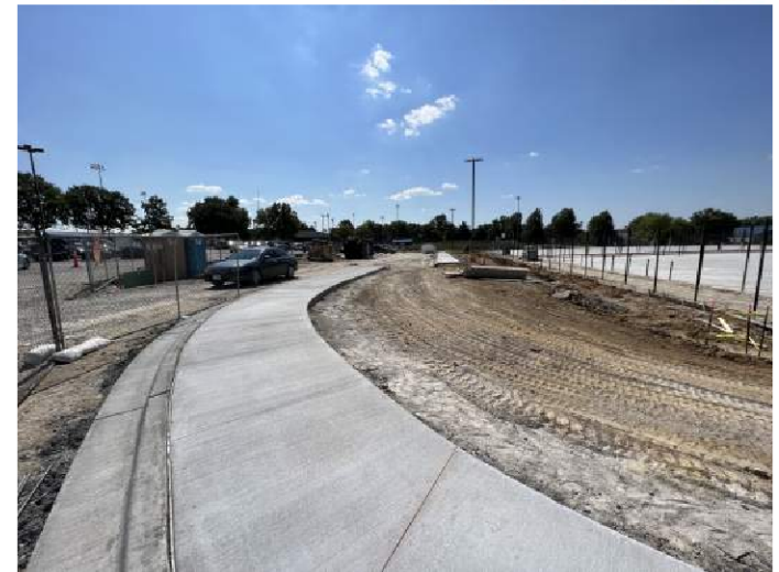
Looking South Curb and Sidewalk
