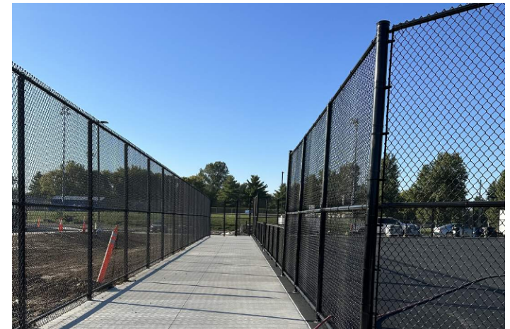
East Concourse Looking South
