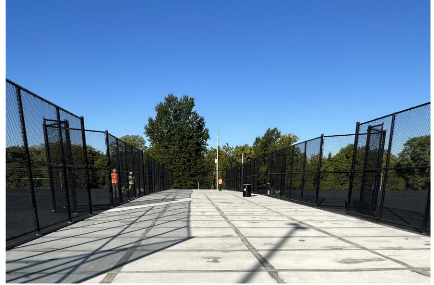
Center Spectator Area Surfacing Prep - Looking West
