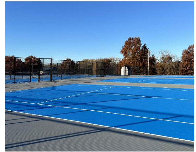
North Courts Looking Southwest
