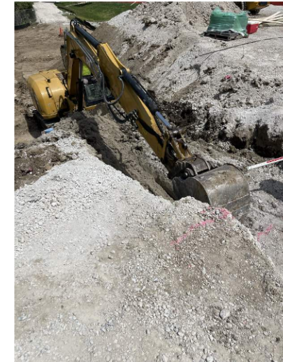
EPiC Elementary - Digging Footings
