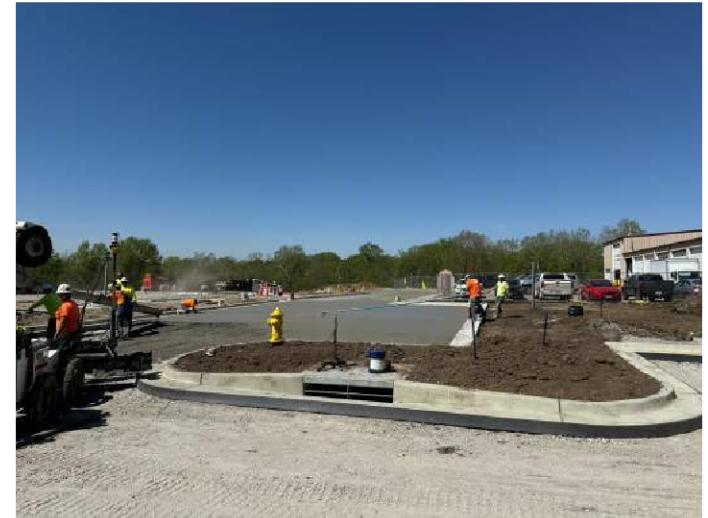
Pouring New Drive at North Entrance
