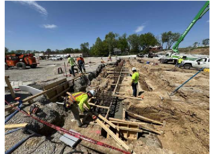
Footing at Southeast Corner of Building
