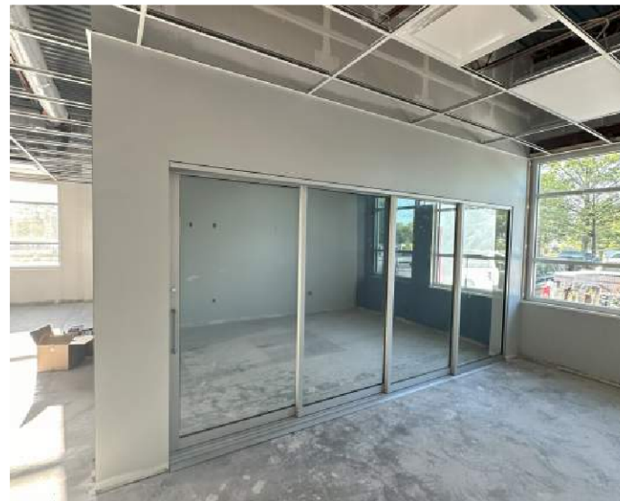
Sliding Glass Wall in Fine Arts Open Office
