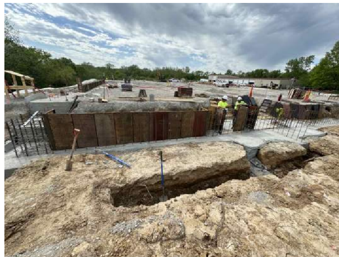
Footing at Southeast Corner of Building
