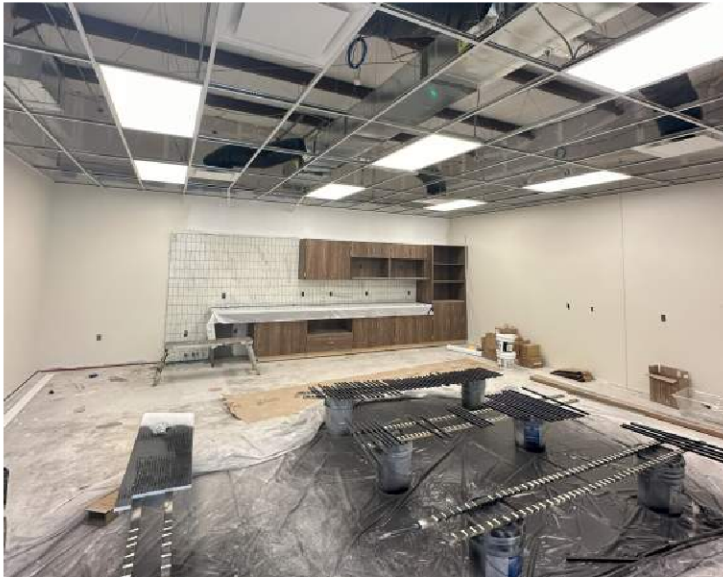
Break Room Casework and Tile
