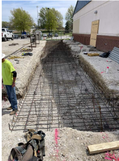
EPiC Elementary - Footing Prep
