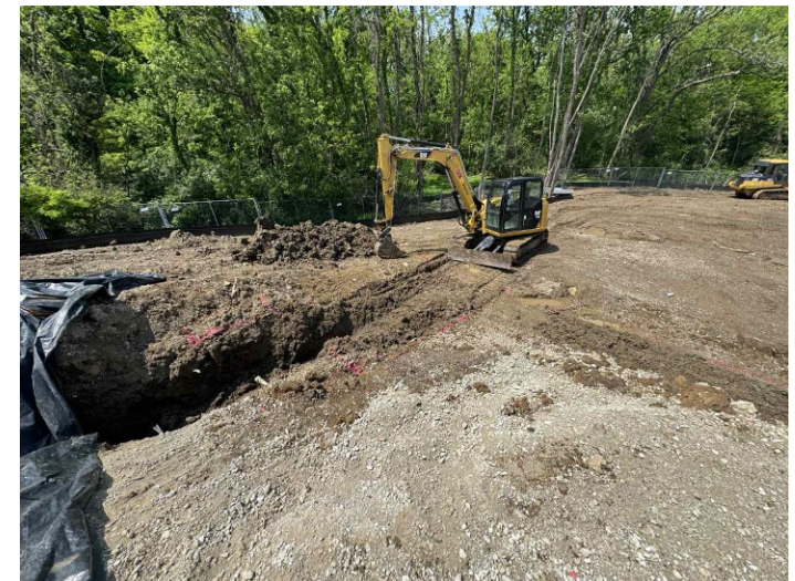
EPiC Elementary - Digging Footings
