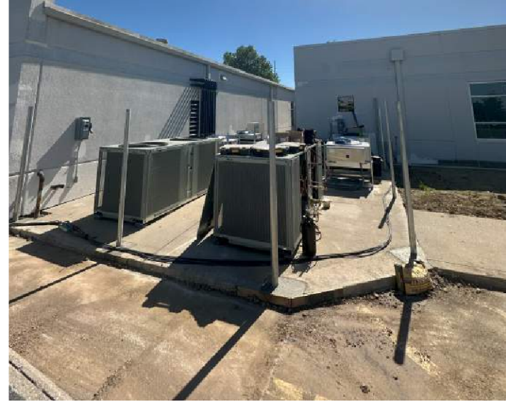
HVAC Equipment Install
