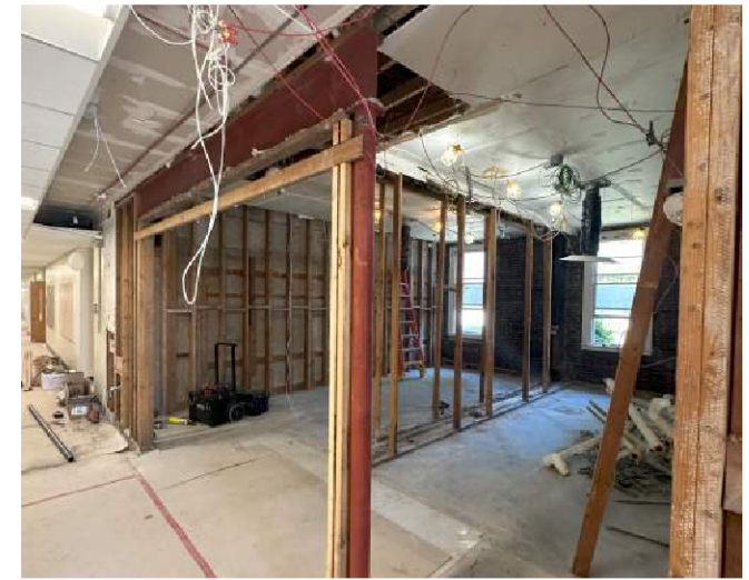
Franklin - Restroom Demolition
