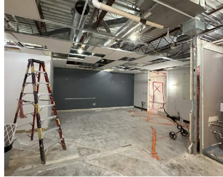
Doniphan - Teacher's Lounge Demolition
