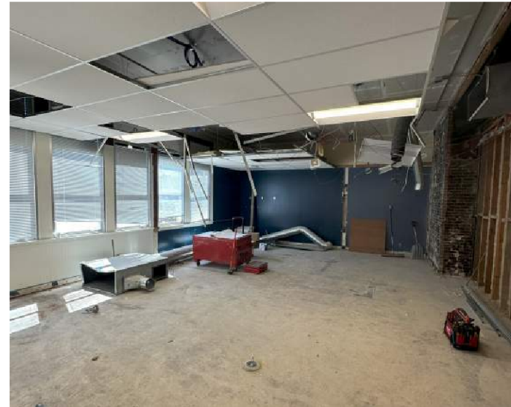
Franklin - Admin Office Demolition
