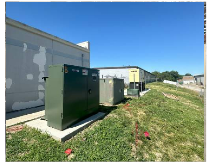
Transformer and Generator Install
