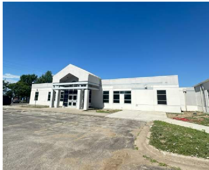
District Tech Center Exterior
