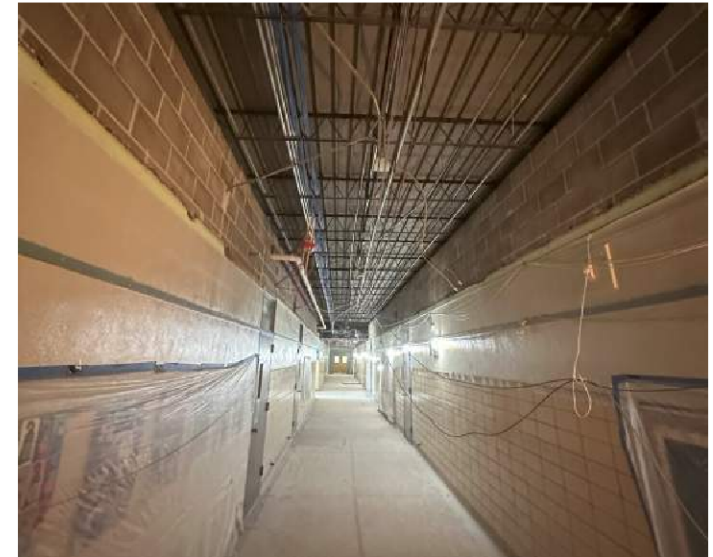
Ridgeview - Hallway Ceiling Demolition
