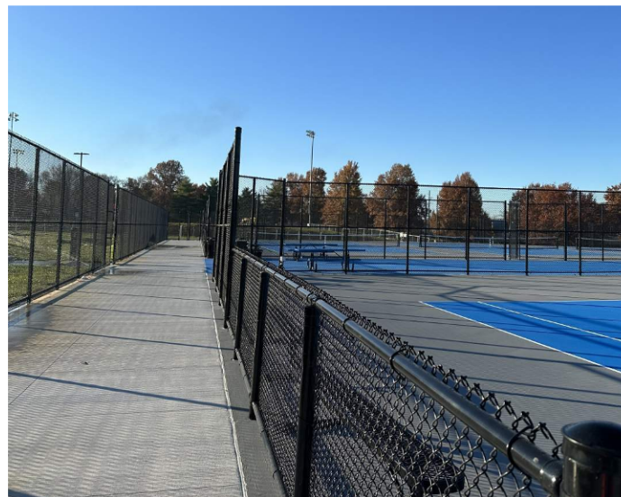
East Concourse Looking South
