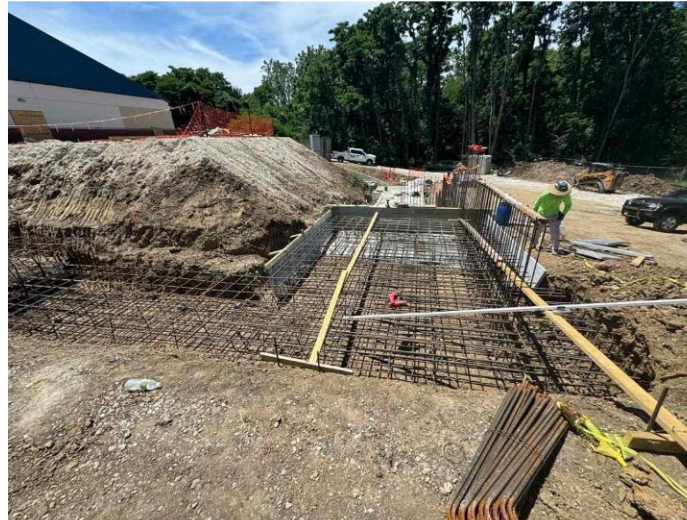
EPiC Elementary - Footing Prep
