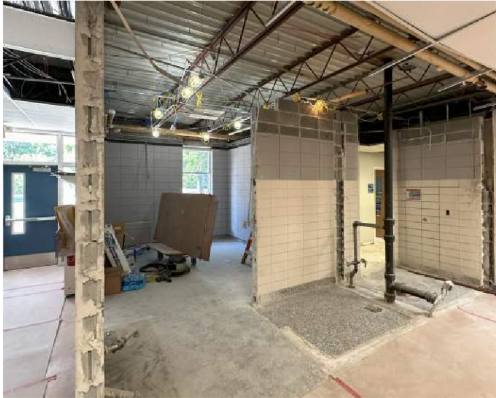
Doniphan - Nurse's Office Demolition
