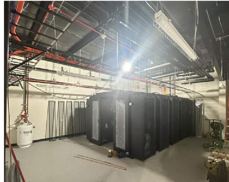
Data Pod Install
