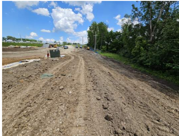
South Entrance Deep Fills
