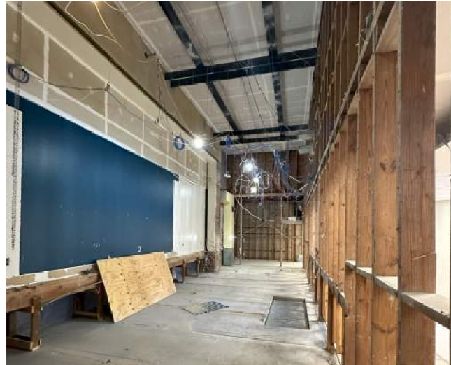
Franklin - Stage Demolition
