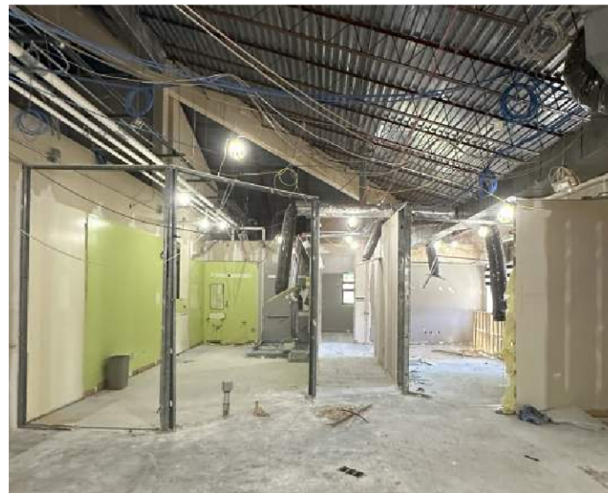
Ridgeview - Admin Office Demolition
