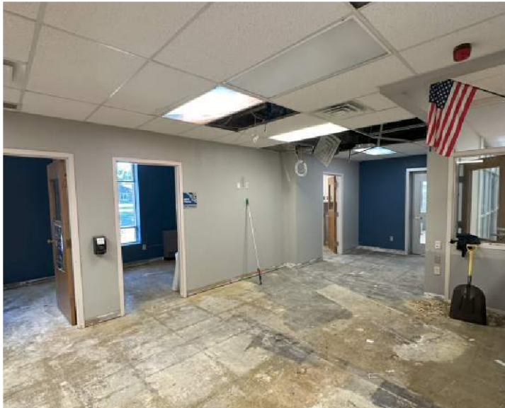
Doniphan - Admin Office Demolition
