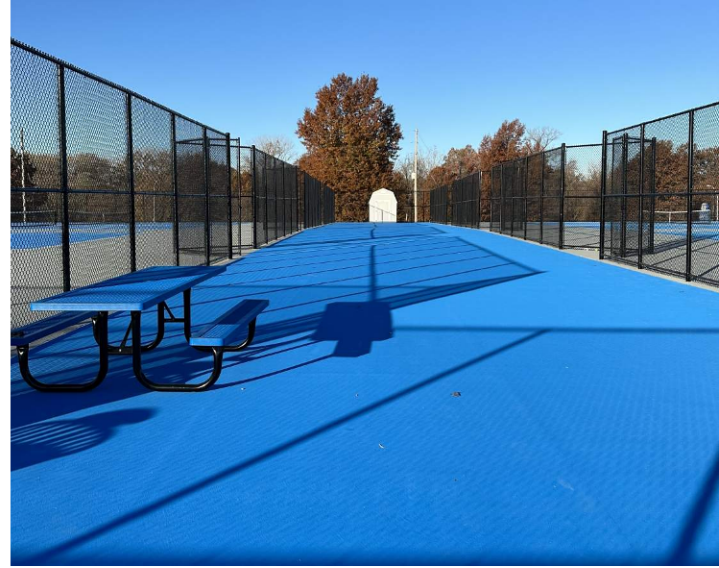
Center Spectator Concourse Looking West
