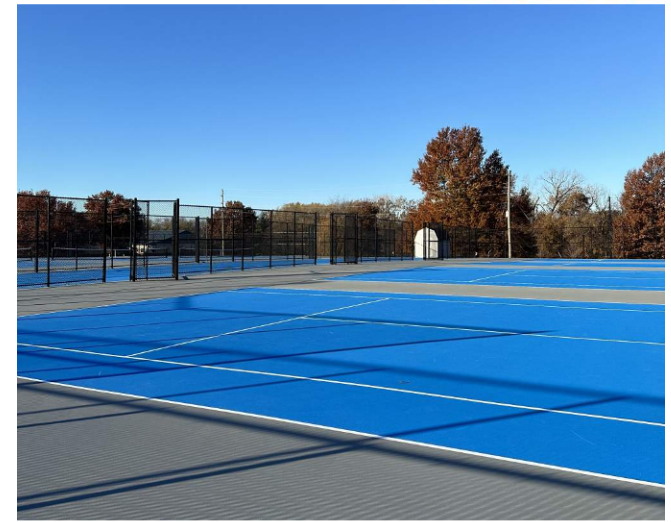
North Courts Looking Southwest
