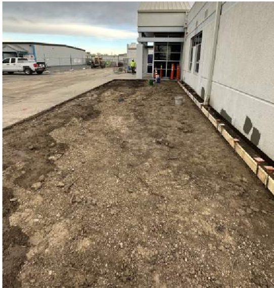
District Technology Center
