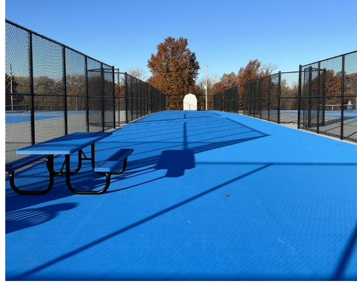
Center Spectator Concourse Looking West
