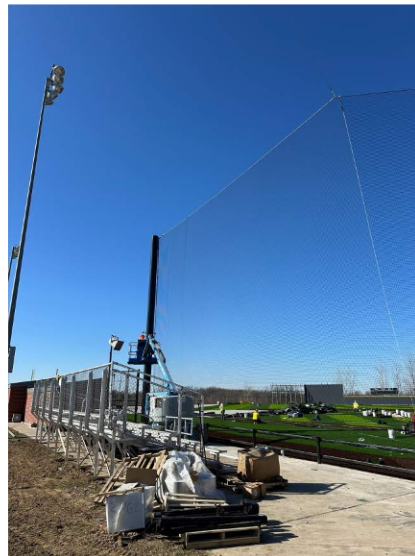
LNHS - Baseball (Backstop Netting Installed)
