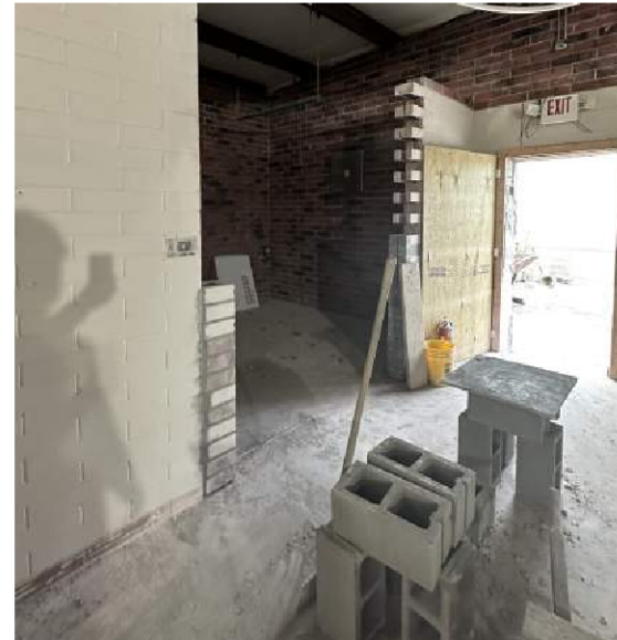
District Technology Center
