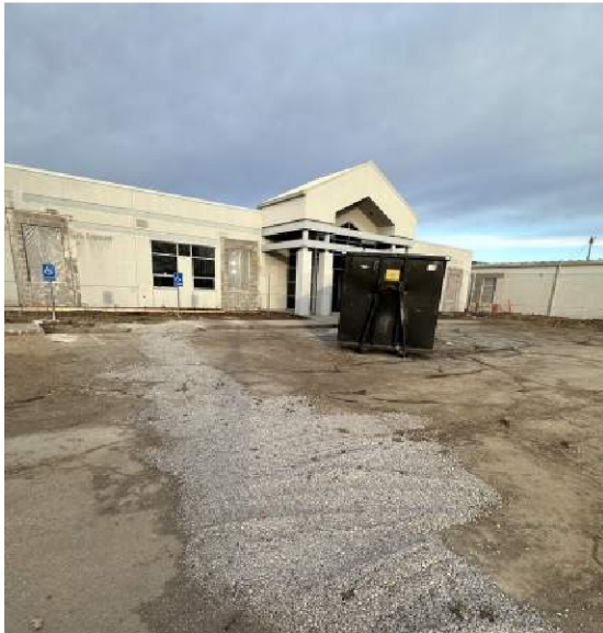
District Technology Center
