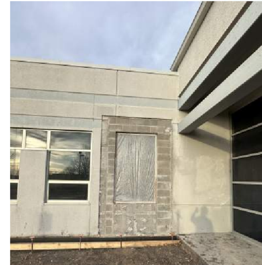
District Technology Center
