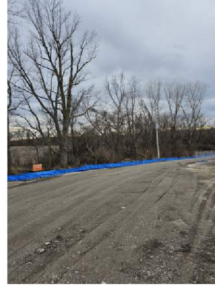
Temp Road (Asphalt Millings)
