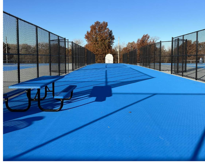
Center Spectator Concourse Looking West
