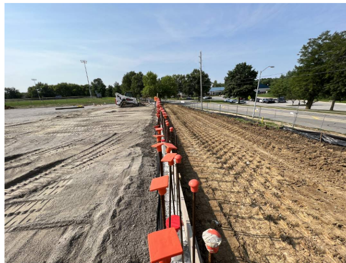
Looking South at Wall
