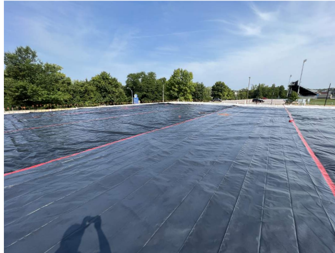
North Court Vapor Barrier for PT Slab
